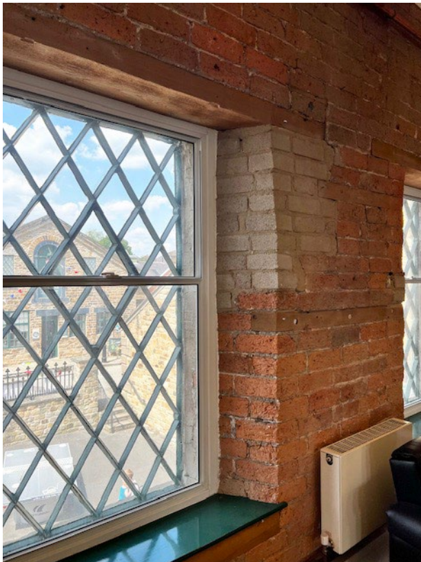
Proposed blockwork removal and brick restoration location (on Southern elevation):
