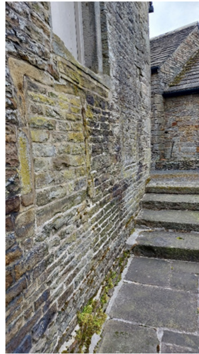
Stone mullions and headers remain of two stoned in windows
