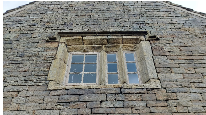
Upper floor stone mullioned window
