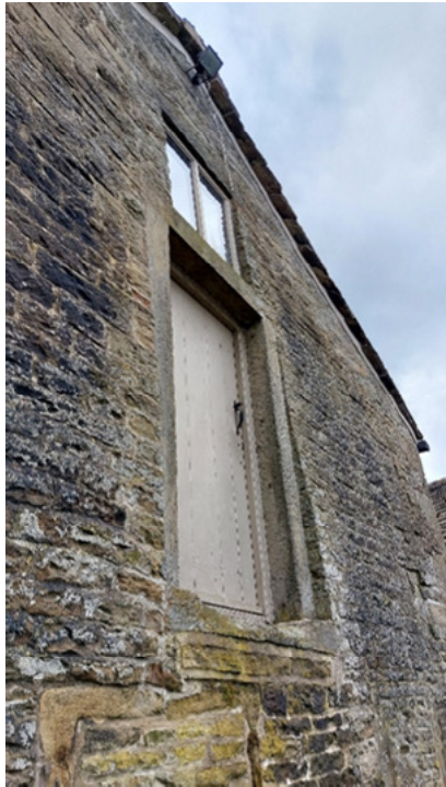
Stone mullioned upper floor door with window above
