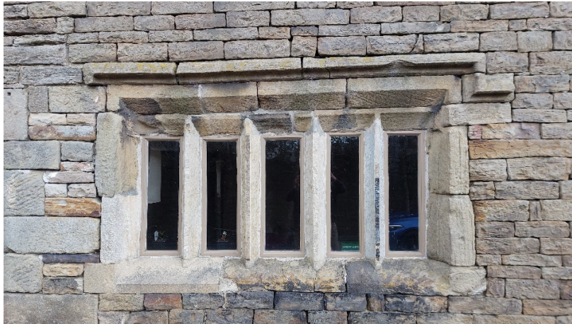
South elevations, ground floor stone mullioned windows with hooded mouldings
