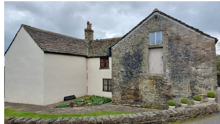
Rear (north elevations)
