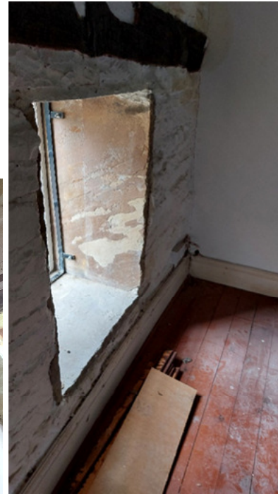
Stone surround to side window
