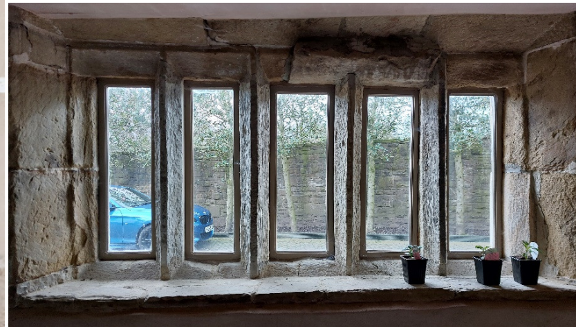
The stone detailing remains internally
