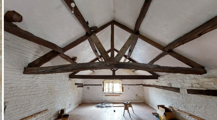
Upper floor king post trusses, this truss to the south has historically been replaced, possibly when the roof was raised, the others it is assumed are original. The walls are whitewashed stone, the floor is a more recent suspended timber with floorboards
