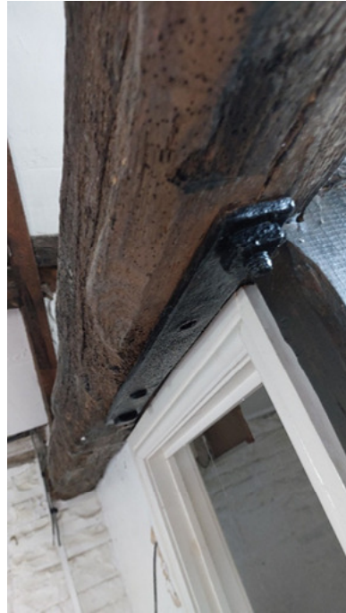
Steel plate to truss
