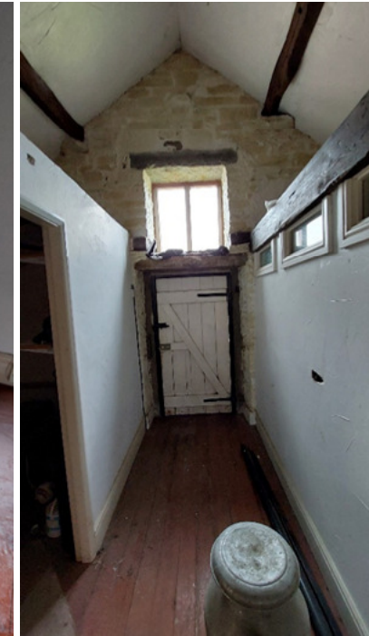
Modern plasterboard partitioning
