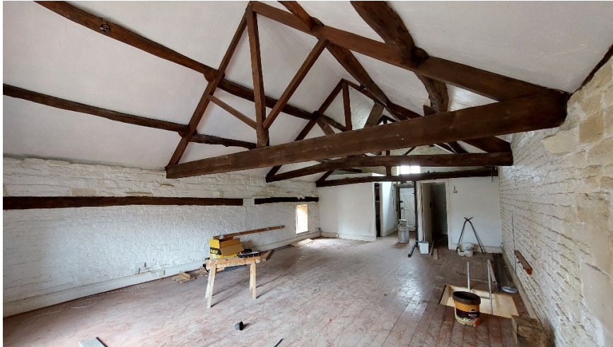
Upper floor king post trusses, this truss to the south has historically been replaced, possibly when the roof was raised, the others it is assumed are original. The walls are whitewashed stone, the floor is a more recent suspended timber with floorboards
