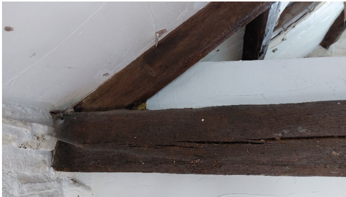
Truss to wall connection
