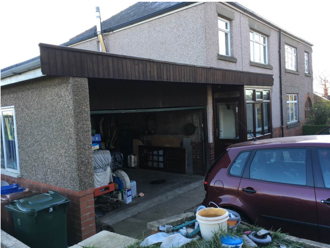
02. Entrance to existing garage – front elevation.
