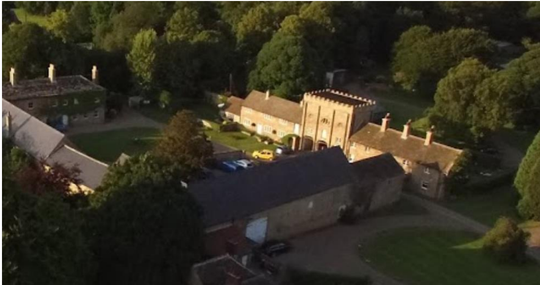
Fig 10 – Hooten Pagnell Hall – Castellated Parapet
