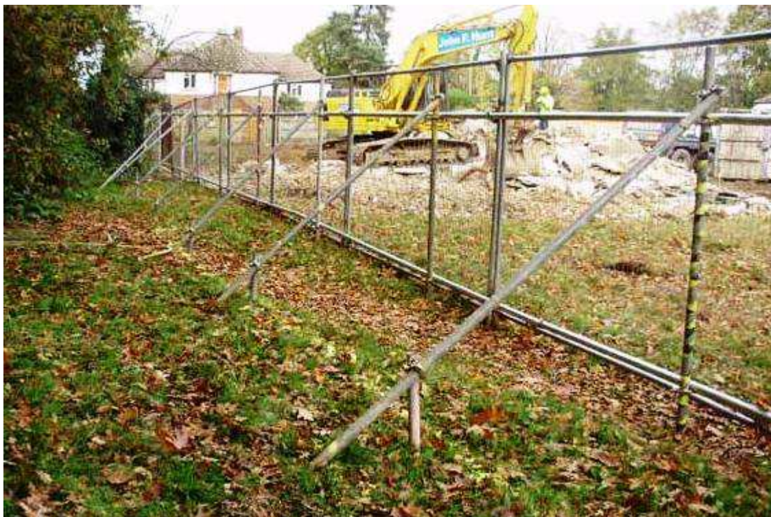
Figure 2: 'Photo of Fencing to BS 5837: 2012'.
