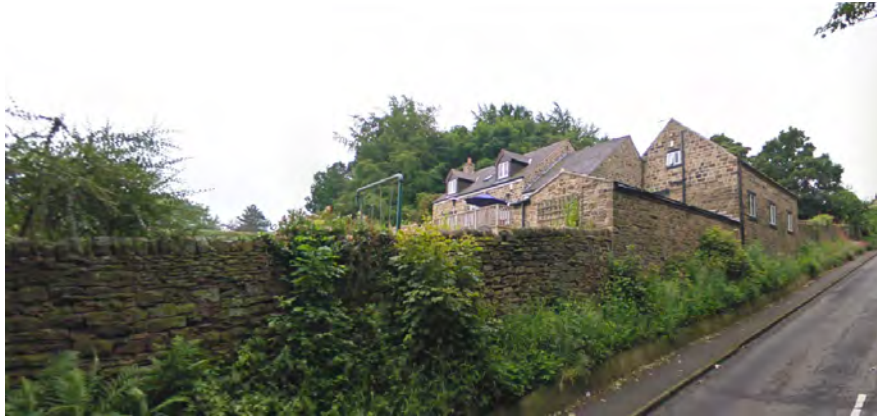
Existing Property From Northeast On Lowe Lane
