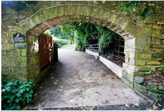
Existing Access Arch And Shared Drive
