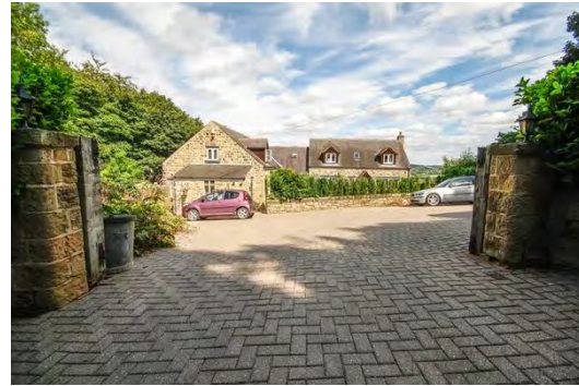
Existing West Elevation From Site Access Gate
