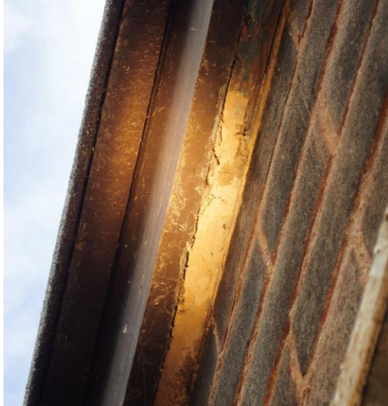
Figure 7 Mortar generally well-sealed behind barge board of brick buildings
