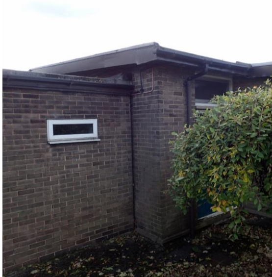
Figure 21 Location of birds' nest in gap between walls (Ward 3 - western aspect)
