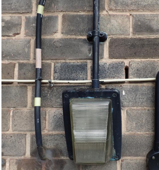
Figure 10 Gap in brickwork on rear of main building, north east of Ward 1
