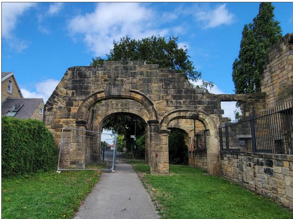
View of the West Gatehouse, looking north
