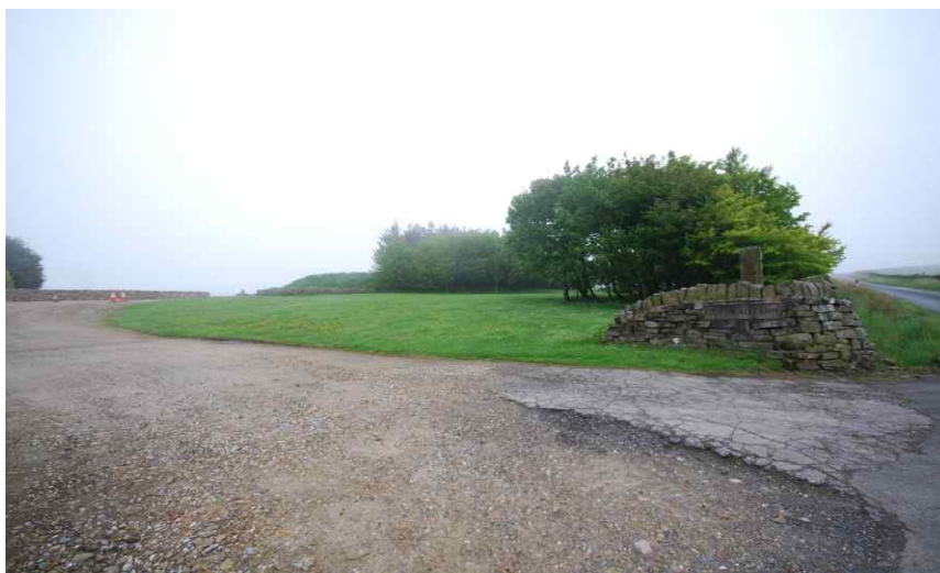
Existing entrance to south side
