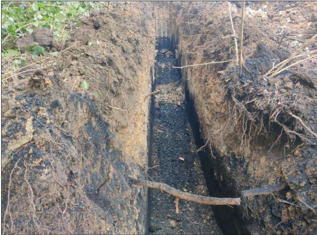
Photo 5: TP02 – Overview of the trial pit.
