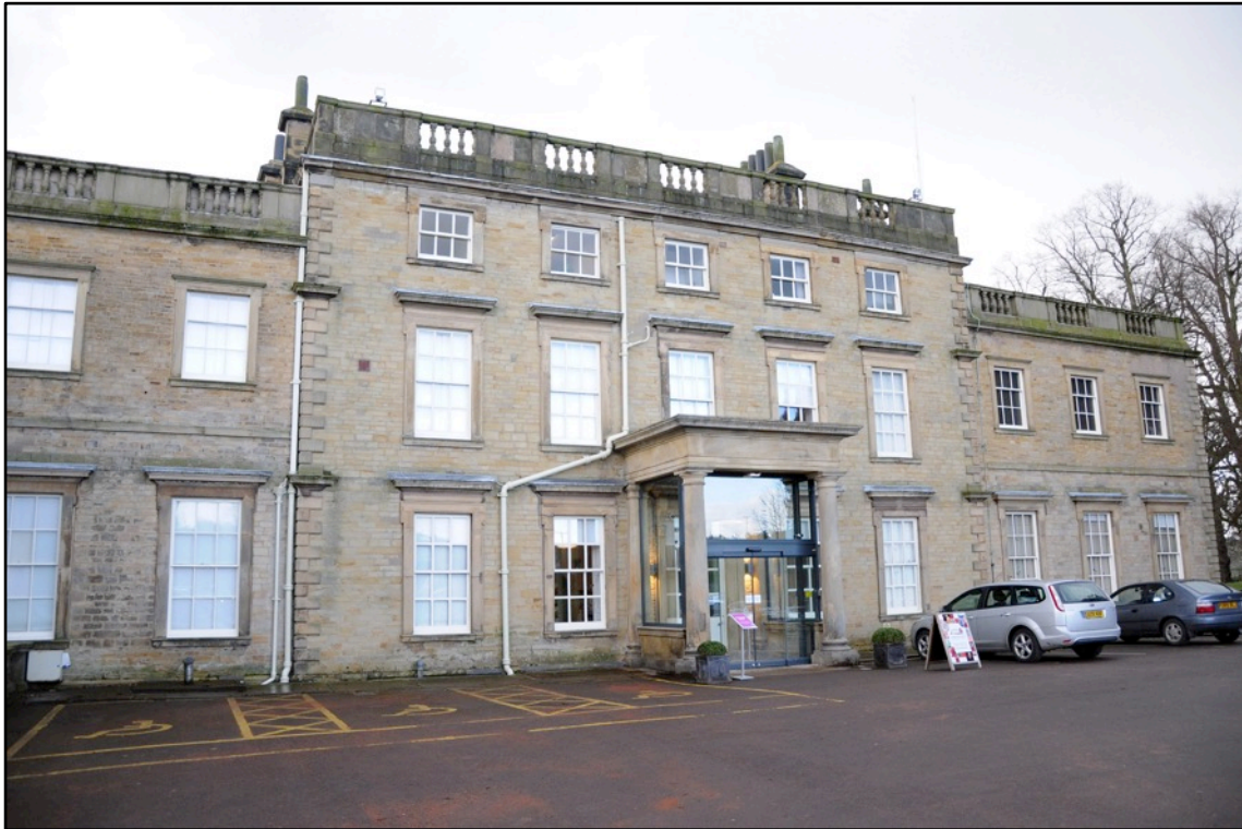
Appendix I.1: General view of external north elevation of Cannon Hall.
