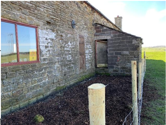
Photo of Lean-to taken from East end facing West
