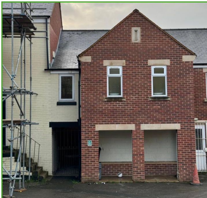
Photo 3: View of Building B2
