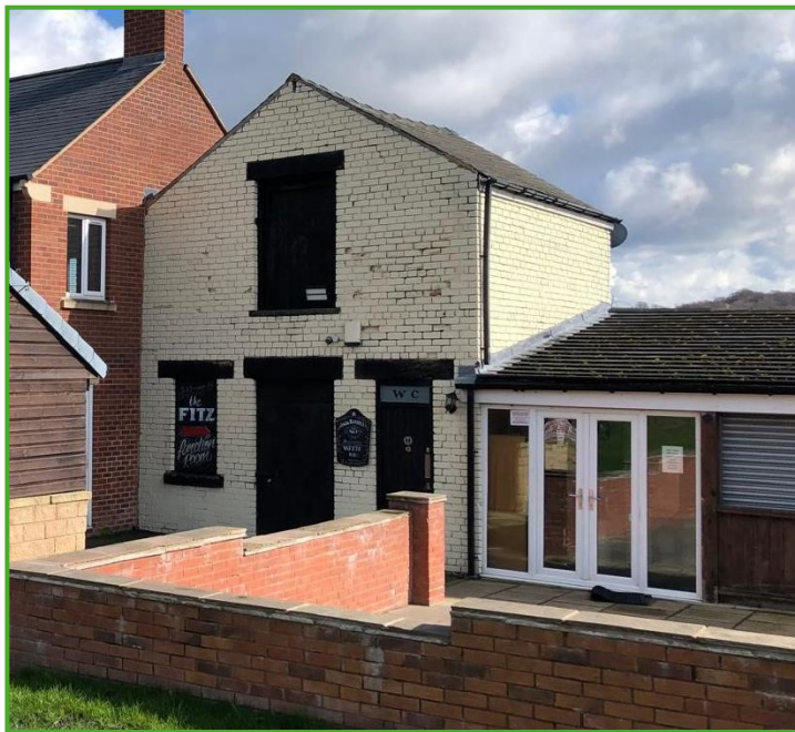
Photo 3: View of Building B3
