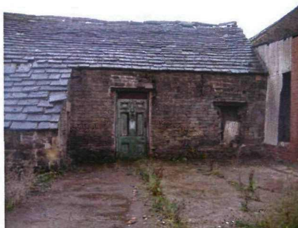
Fig 17 East elevation – Barn B – north end
