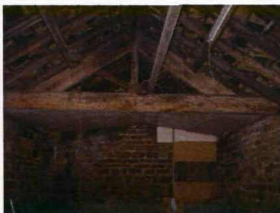
Fig 19 End truss looking west
