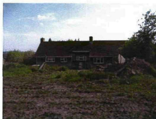
Fig 2 North elevation of bungalow
