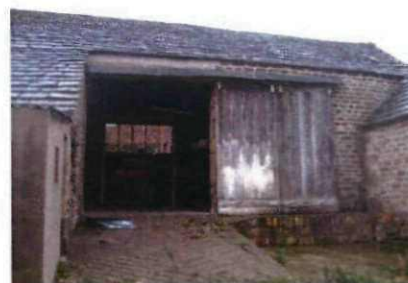
Fig 15 Typical storey height – barn door opening
