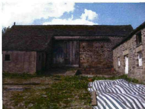
Fig 3 South elevation – Barn A
