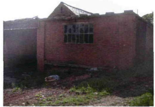
Fig 6 Brick extension to NE corner - Barn A
