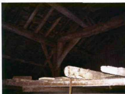
Fig 13 Barn A roof structure
