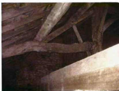
Fig 14 Half truss from timber post
