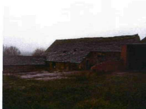
Fig 12 North and east elevation – Barn B
