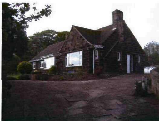
Fig 1 South and east elevation of bungalow
