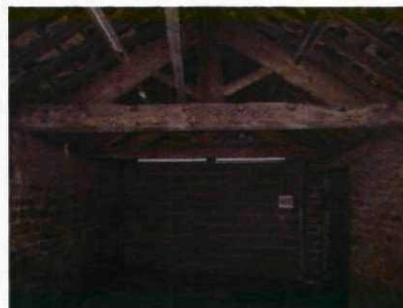
Fig 20 End truss looking east
