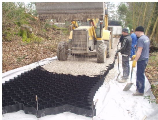
Photo 4- once filled the system can support plant to carry aggregate to the fill area
