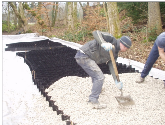
Photo 3- expanding and filling the Cellweb system
