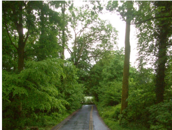
Photo 5- completed road using porous tarmac surfacing
