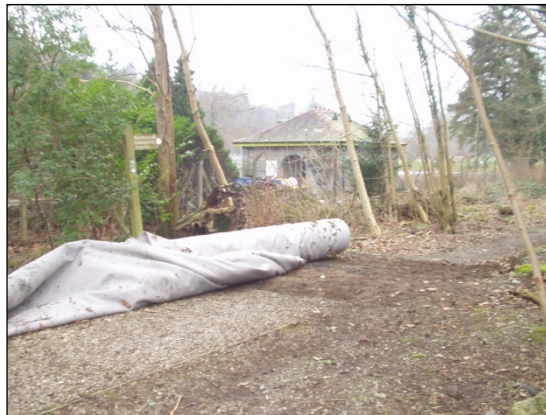
Photo 2- laying of Fibretex material onto existing subgrade
