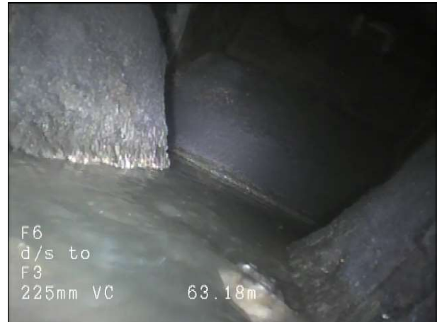
Photo: 7_7A 63.2m, Finish node type, manhole reference number: F3
