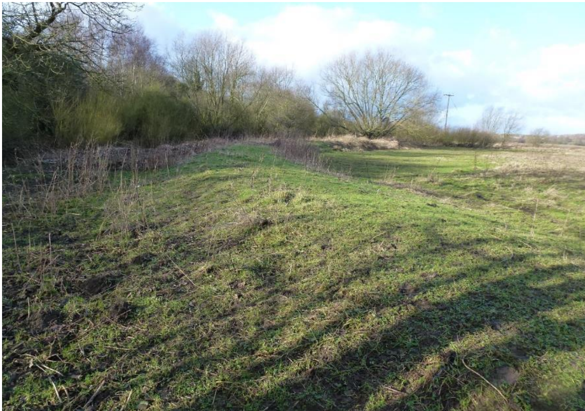
Figure 1-3: Flood Defence on Site
