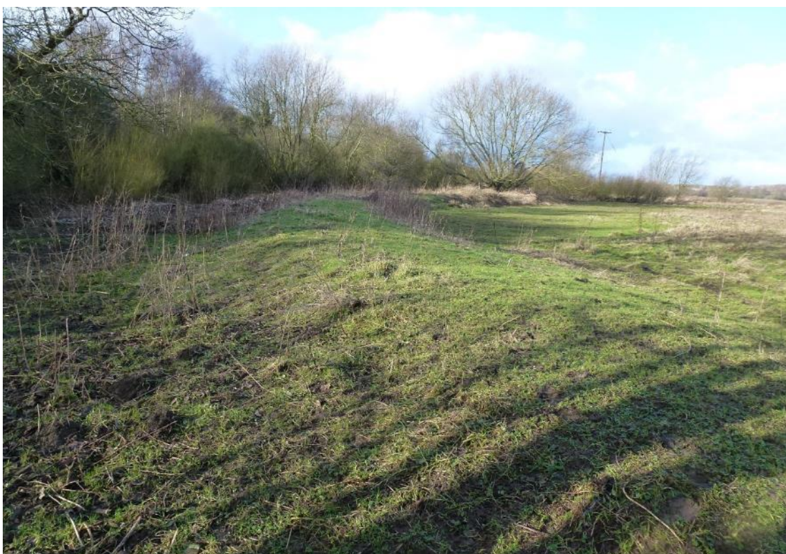
Figure 2-5: Left bank flood embankment to the southwest of the site
