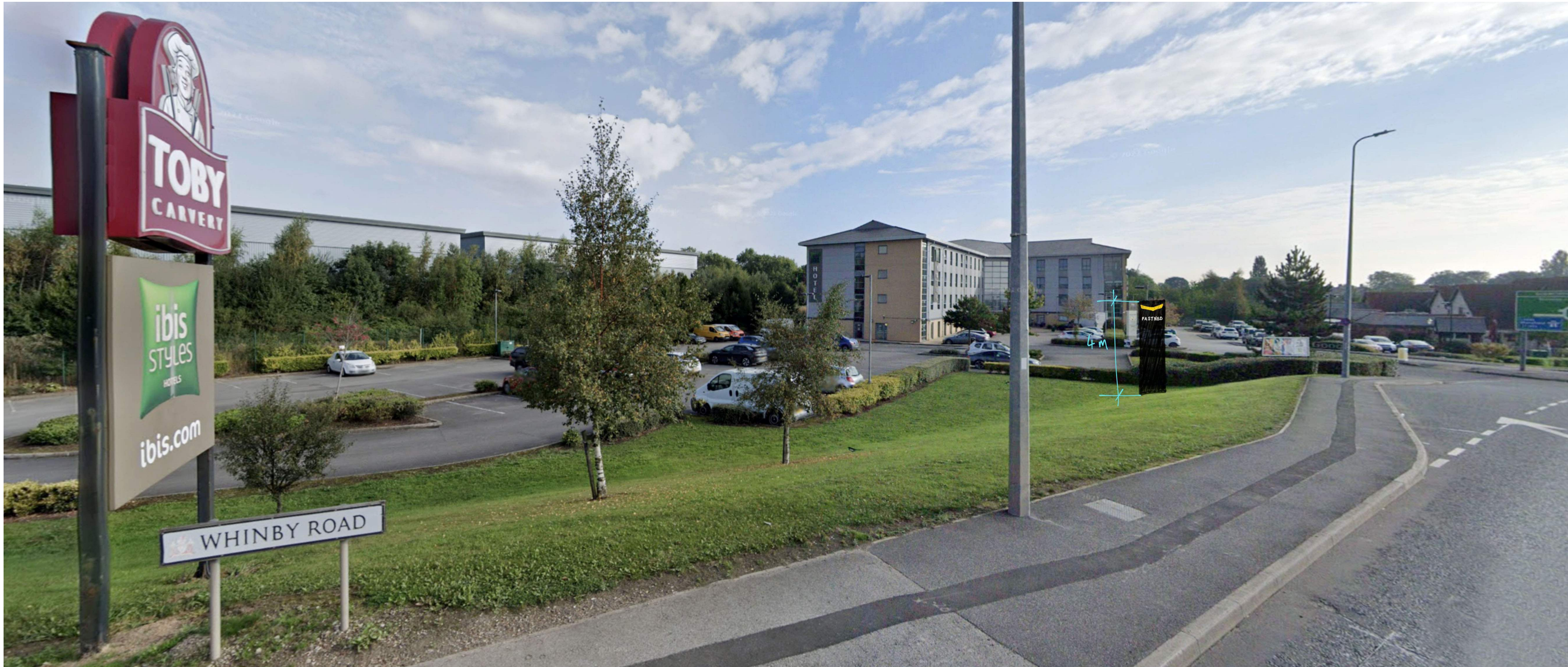
Street view showing totem - ground level below pavement level
