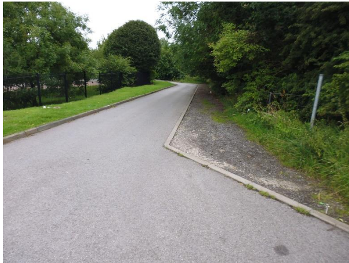
Photo 6: Pedestrian Infrastructure on St Helen's Boulevard (East of Access)
