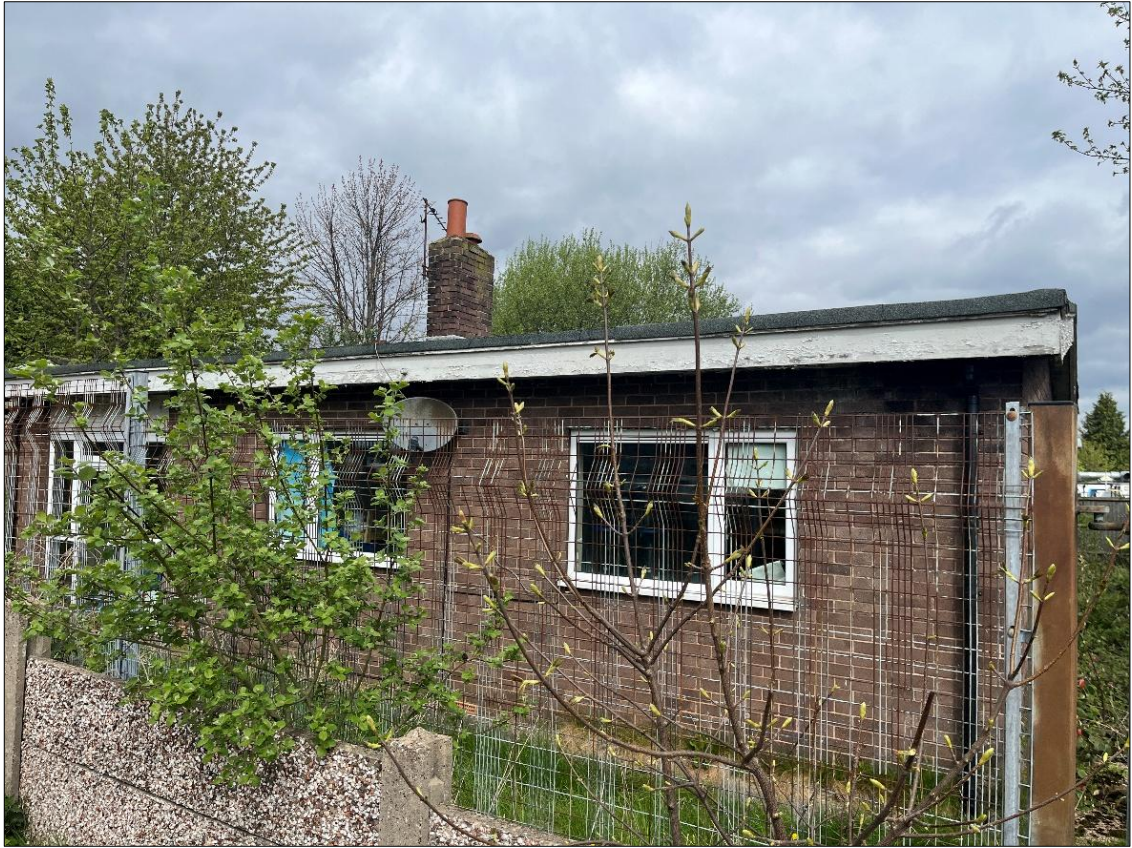
Figure 2: Building 1 on site, fenced within the area of vegetated garden.
