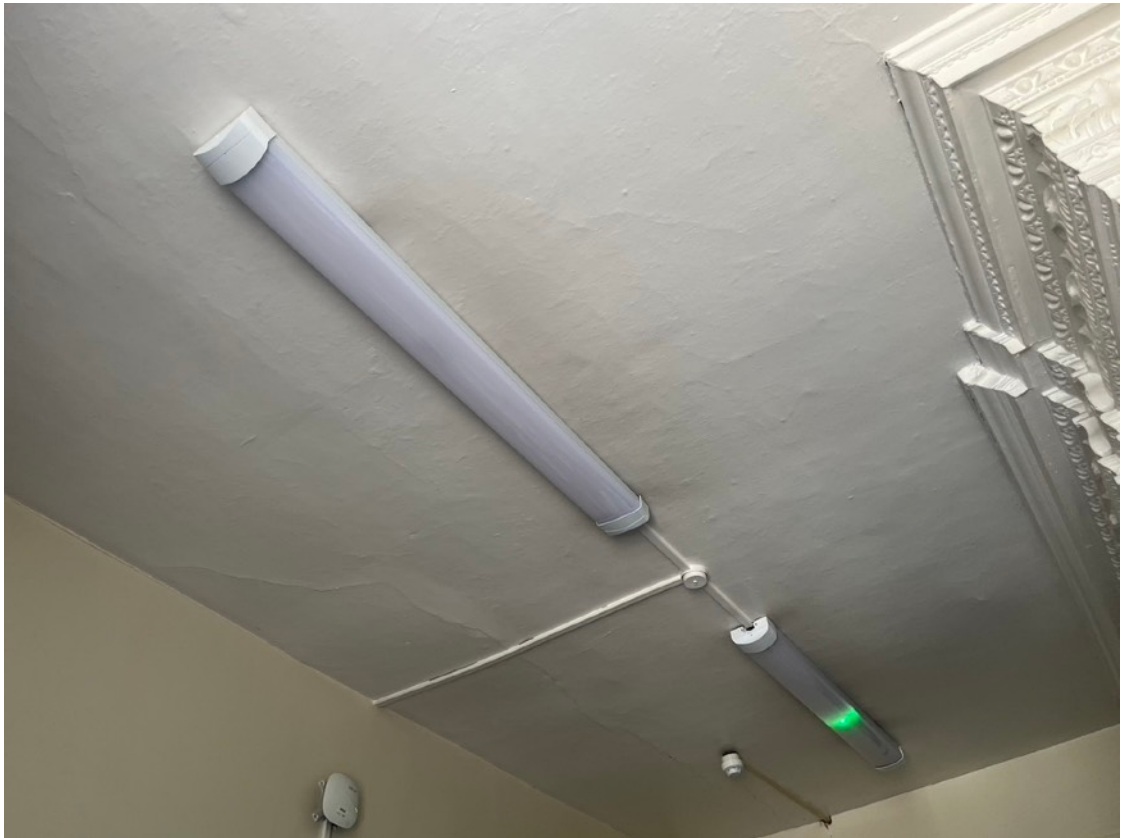
Ceiling office west of C3 showing luminaires to be reused.
