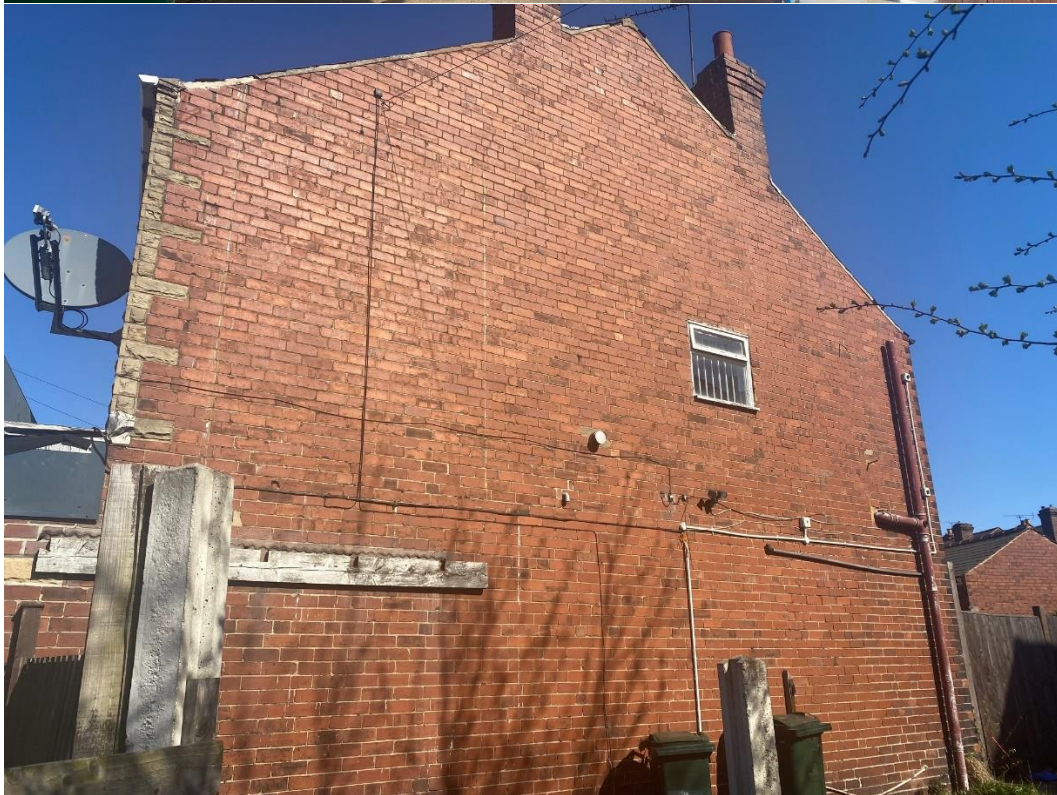
Photo 2 (southern side elevation)
