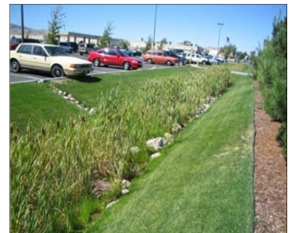
Figure 6-6: Indicative one way cross fall design (left) and constructed vegetated swale (right)
