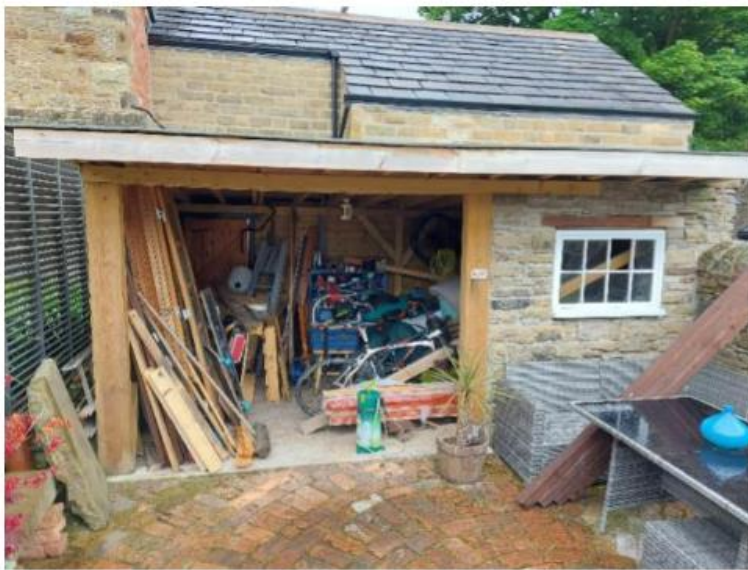
Outbuilding as stands; extension to the left of the original structure, constructed from timber.
