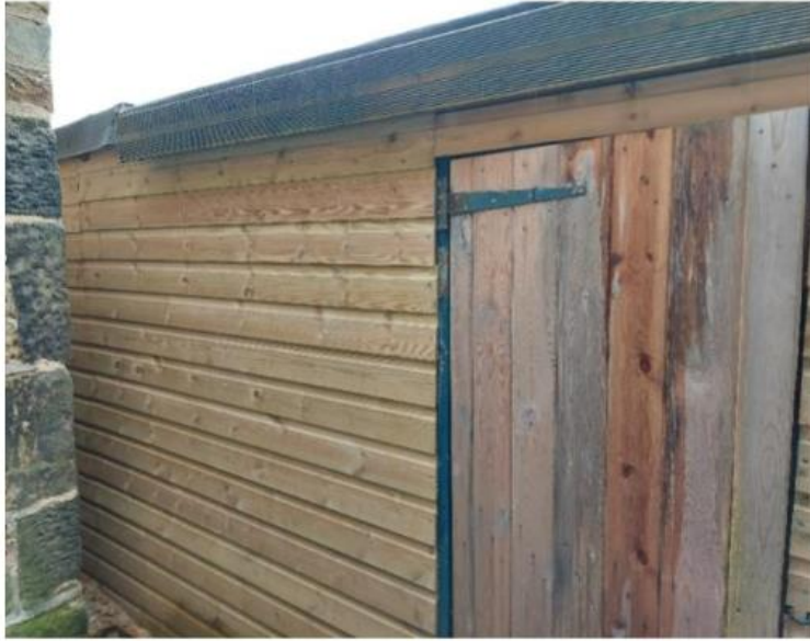
View to the rear of the extension.
