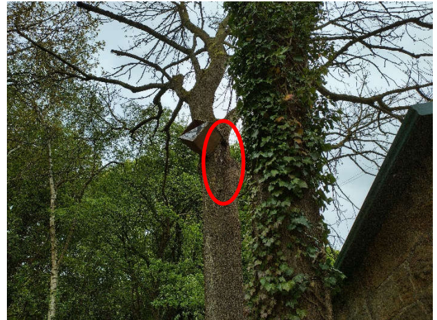
Photo 2: Signs of fungal infection on Ash T60 (circled). Desiccated fungal bracket was found at the base of the tree
