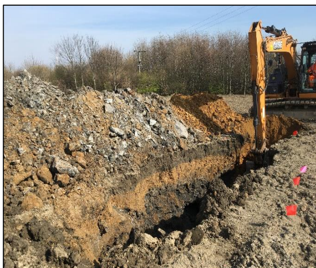
Plate A: View of TT105, with associated arisings. Facing east.
