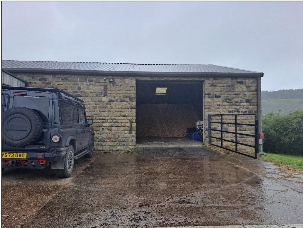
Plate 3-6: View of the eastern end of the barn, where the agricultural storage is located. Photograph taken from the south facing north.
