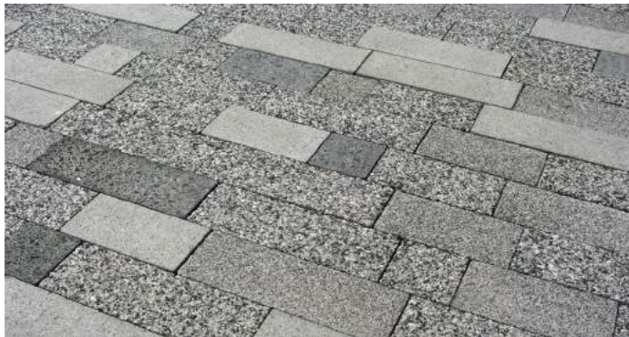
P3 & P4 [demonstrating paving flexibly laid]
