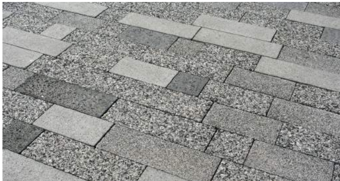
P4 [demonstrating paving flexibly laid]
