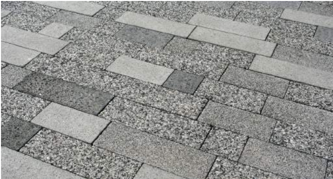
P3 [demonstrating paving flexibly laid]
