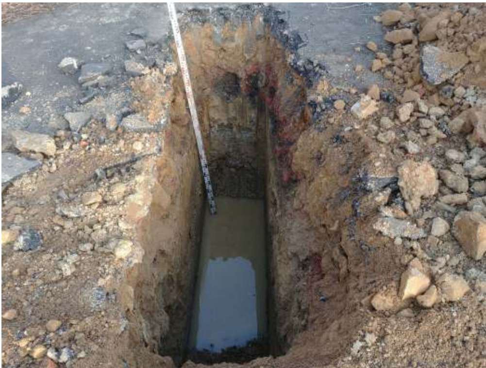
Soil Horizons / Infiltration Testing. TP05.
