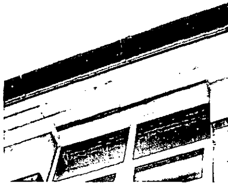
Figure 4: loose soffits at rear of main building
