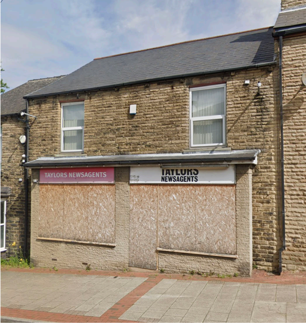
Photograph of Existing Shop front:
