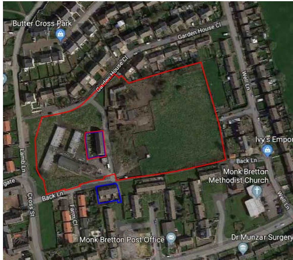
Aerial Photo of Site
