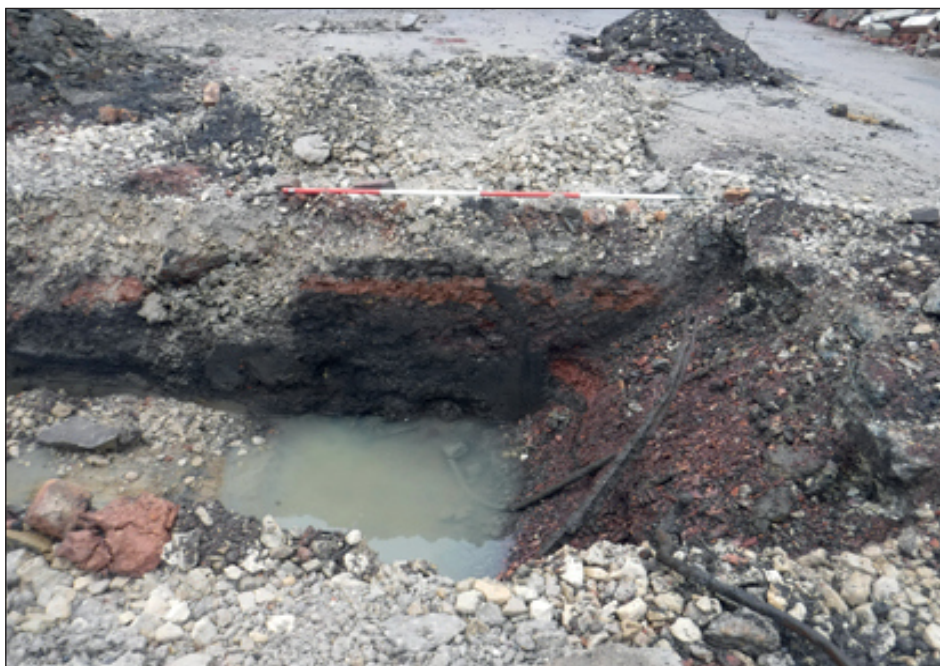
Plate 30. Trench 3: sample section, looking east
