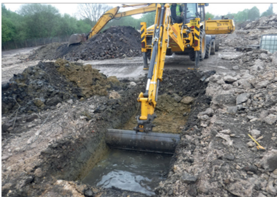
Plate 37: Stripping Trench 4, looking south-west
