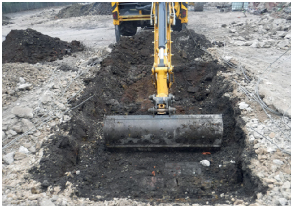
Plate 36: Stripping Trench 4, looking west
