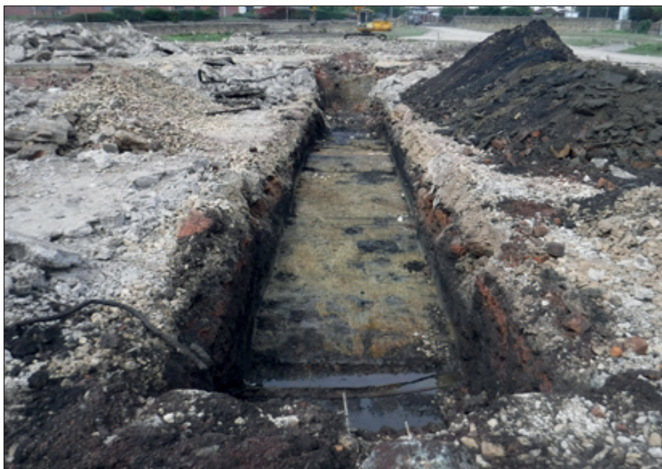
Plate 26. Trench 3, looking north
