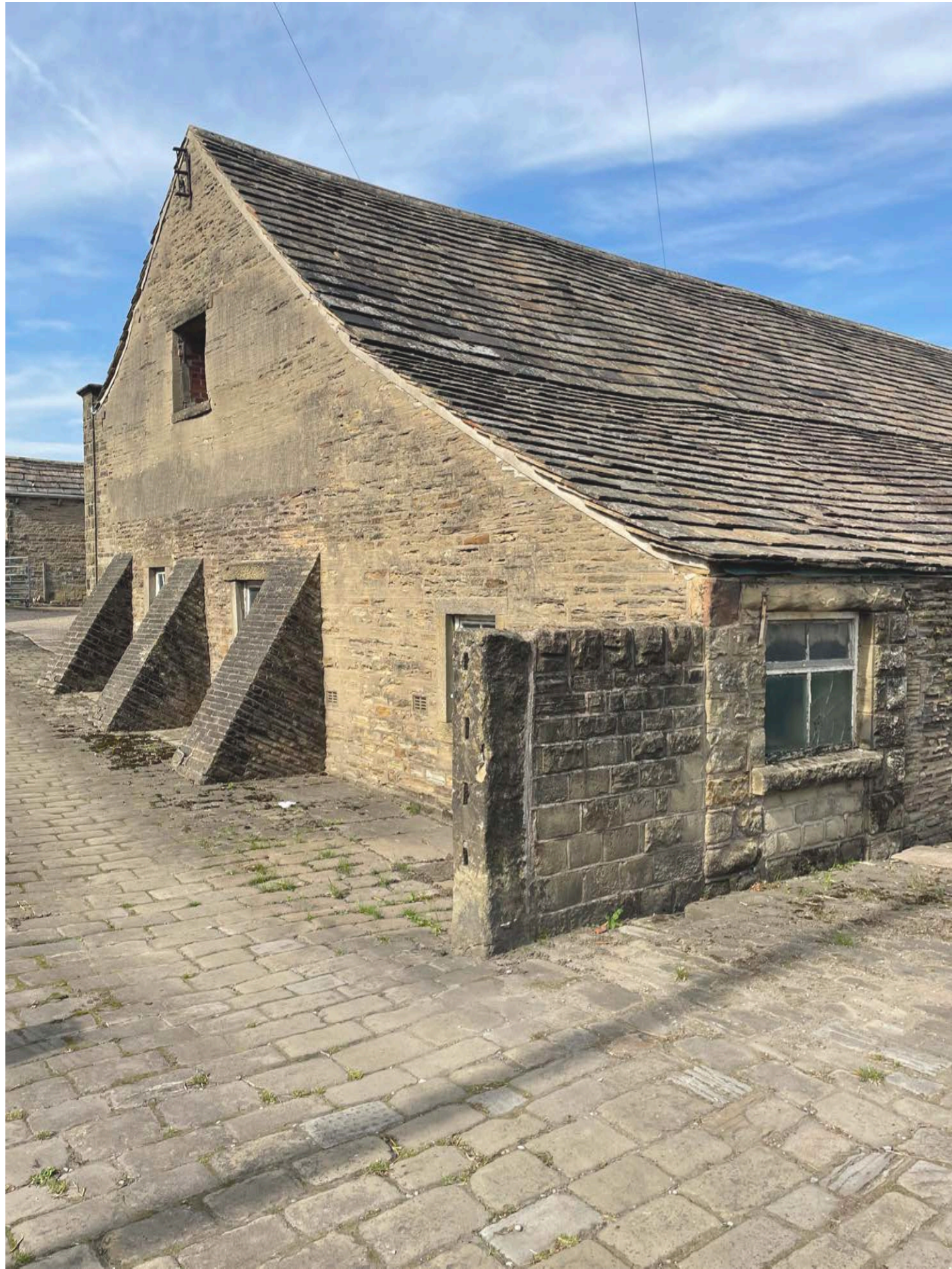
Photo Ref: E04 View of Nether Mill Barn (Side Elevation) from Vehicular Access
