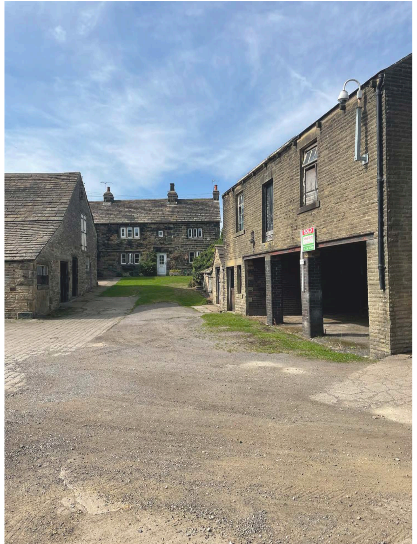
Photo Ref: E05 View of Nether Mill Barn (Side Elevation) from External Area
