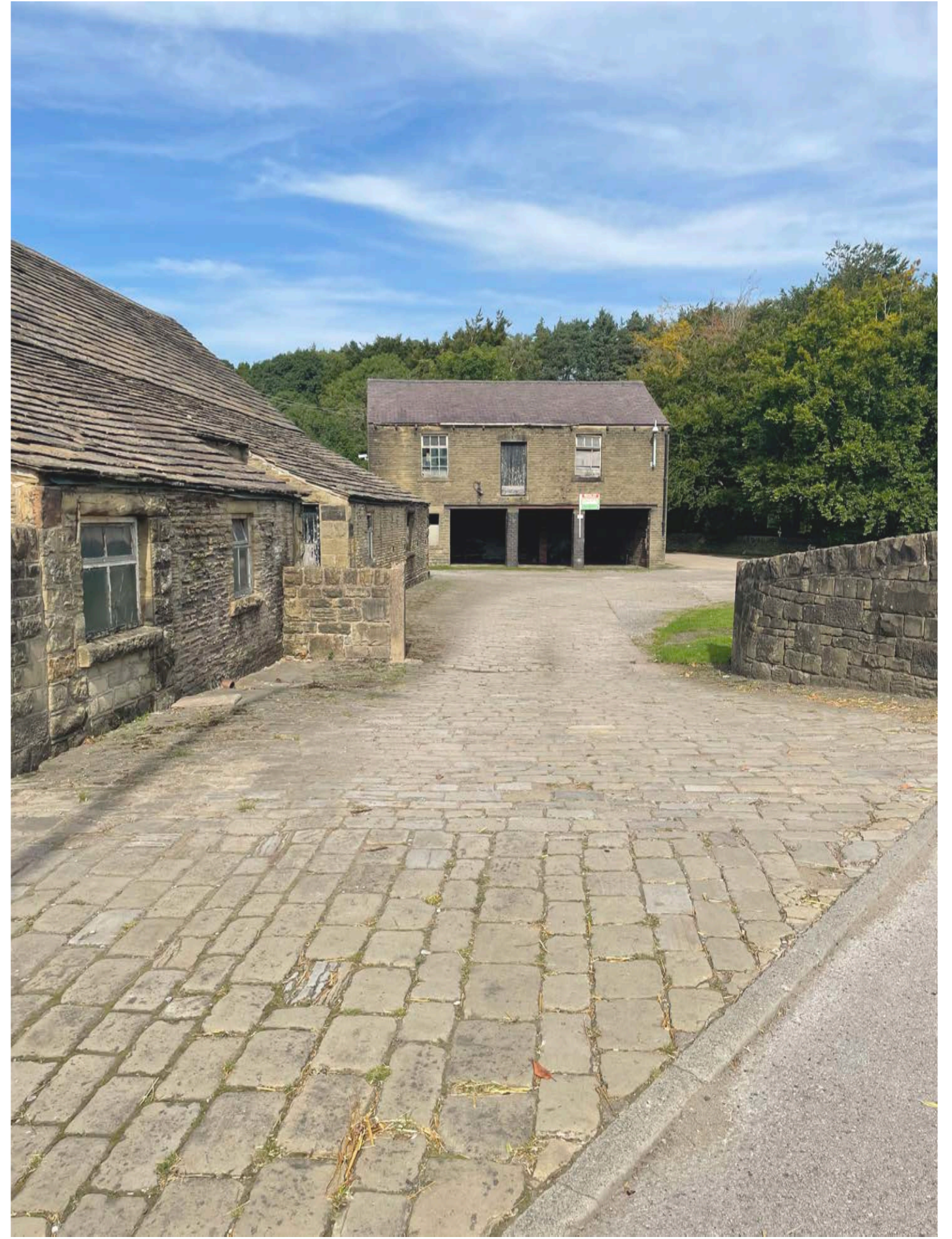
Photo Ref: E02 View from Vehicular Access, Looking North
