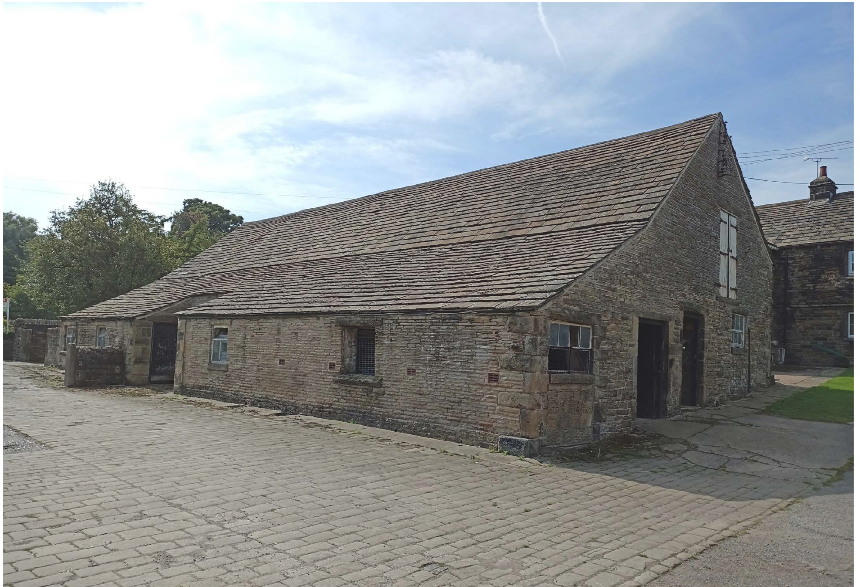
Photo Ref: E03 View of Nether Mill Barn (Primary Elevation) from External Area
