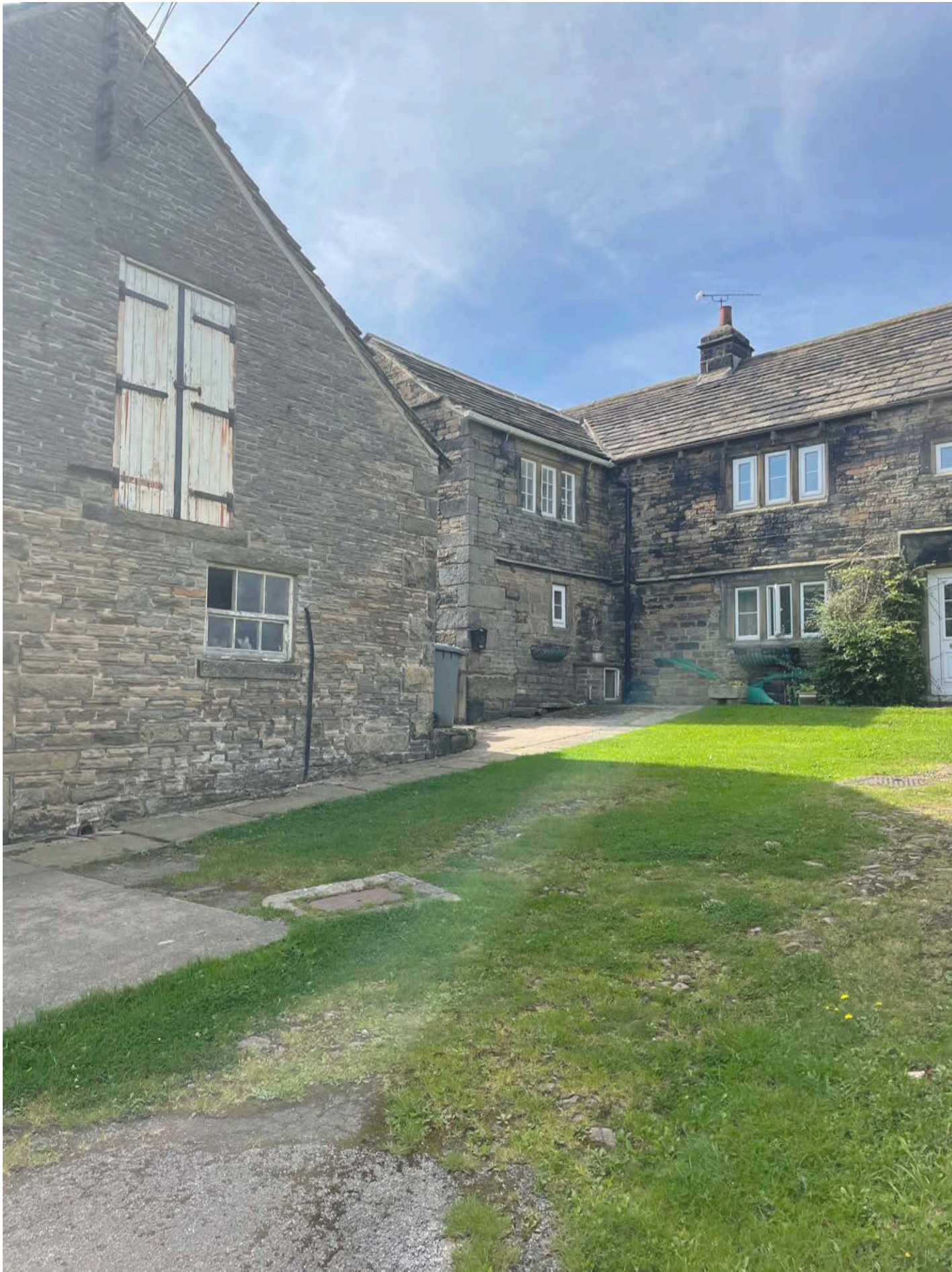
Photo Ref: E06 View of Nether Mill Barn (Side Elevation) indicating relationship with Farmhouse
