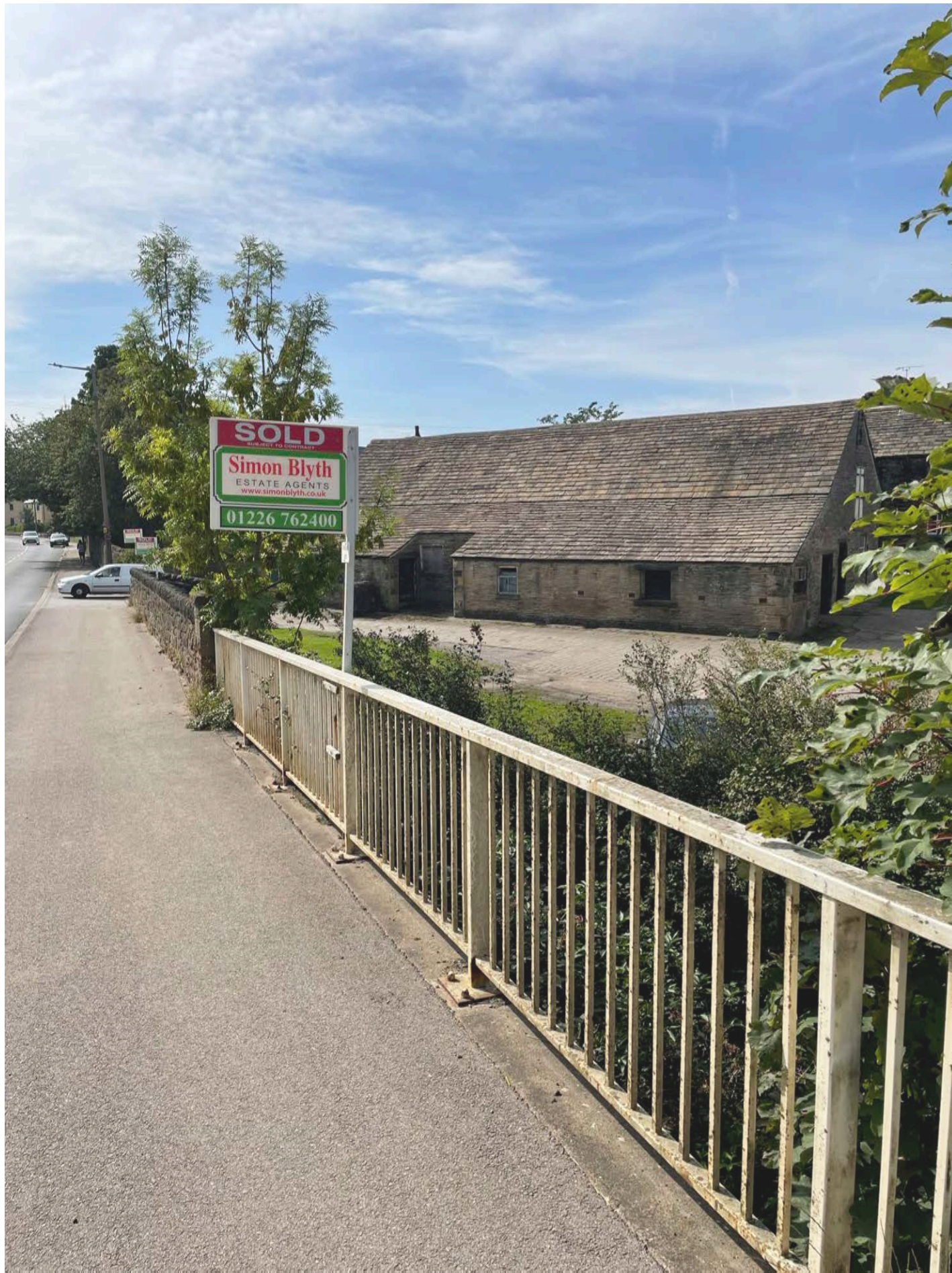
Photo Ref: E01 View from North Eastern Approach, Barnsley Road
