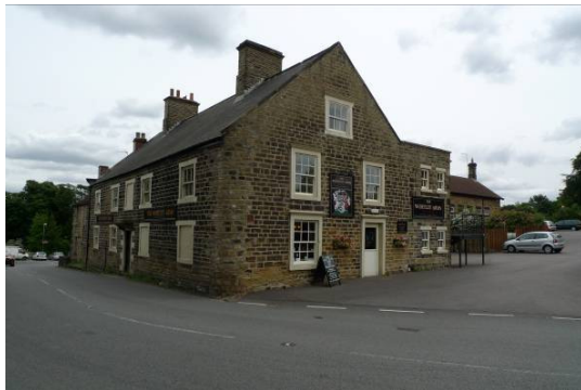
Traditional six pane sashes
