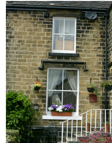
Drip mould over stone lintel
