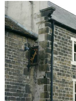
Coursed stone walling with inappropriate struck pointing
