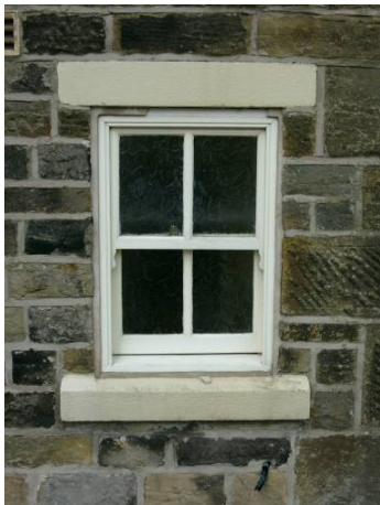
Stone lintel & sill
