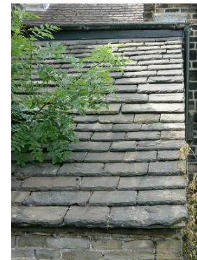
Traditional stone slate roofing
