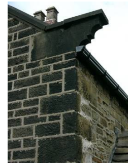
Coursed stone walling with inappropriate struck pointing
