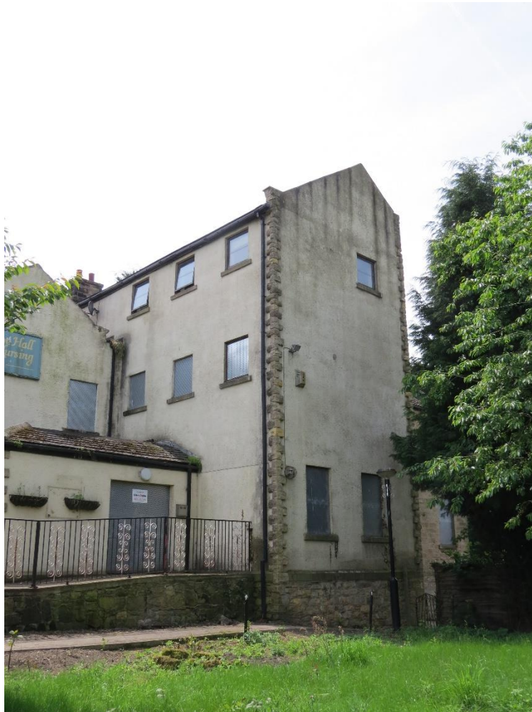
Fig 2: North Elevation, showing late '80s 3 storey extension in rendered masonry.
