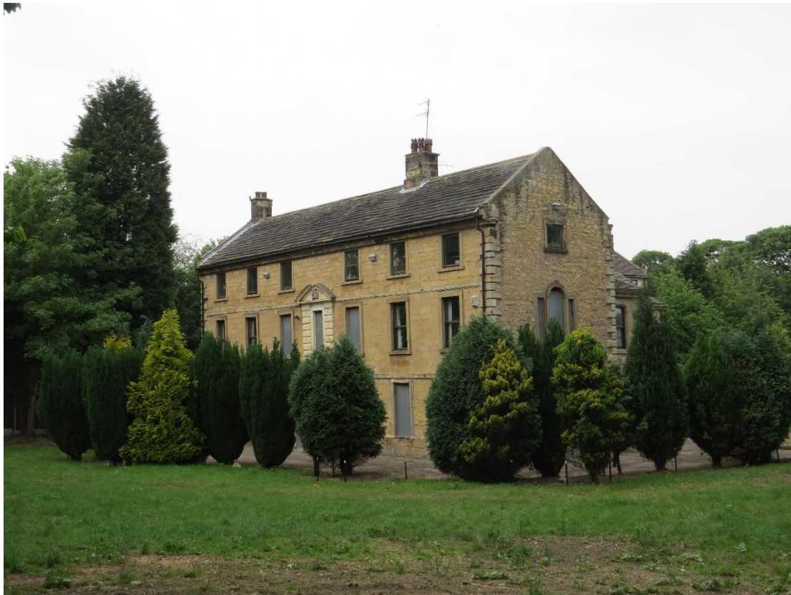
Fig 1. View of south elevation
