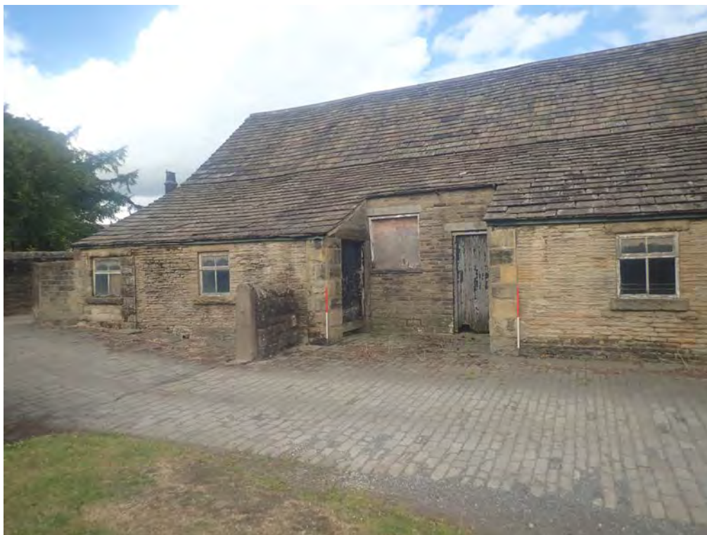
Photograph:2 Direction: W Digital Ref: NEMB2_0004 Description: SW extent of SE elevation detailing SW outshut (left), catslide roof, blocked door at SW extent (left), stone wall, and two doorways.
