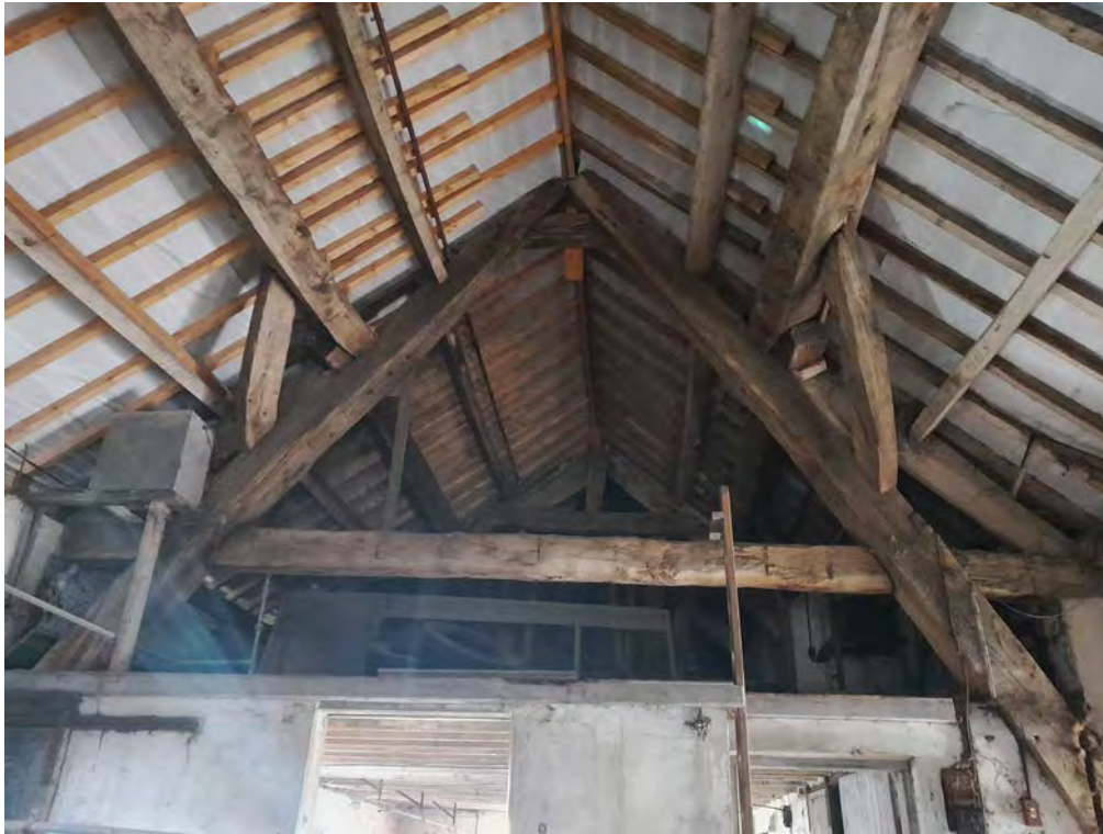
Photograph:29 Direction: NE Digital Ref: NEMB2_0079 Description: General view of SW face of Truss 2 with Truss 3 in background.
