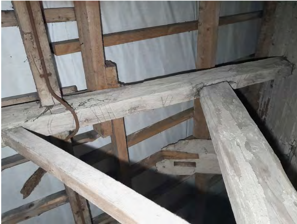
Photograph:67 Direction: SW Digital Ref: NEMB2_0107 Description: Baltic marks in rafter soffit of NE truss of NE outshut.
