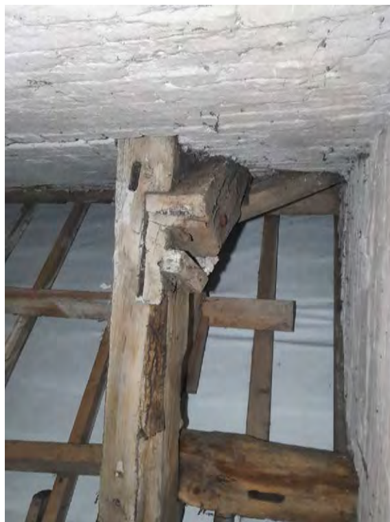
Photograph:47 Direction: SE Digital Ref: NEMB2_0111
