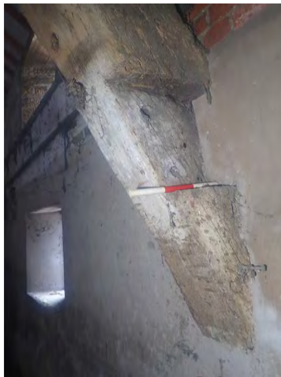
Photograph:30 Direction: W Digital Ref: NEMB2_0037 Description: Detail of 0.3m height of former rail mortice with holes for two former pegs. Internal white paint or discoloration of timber.
