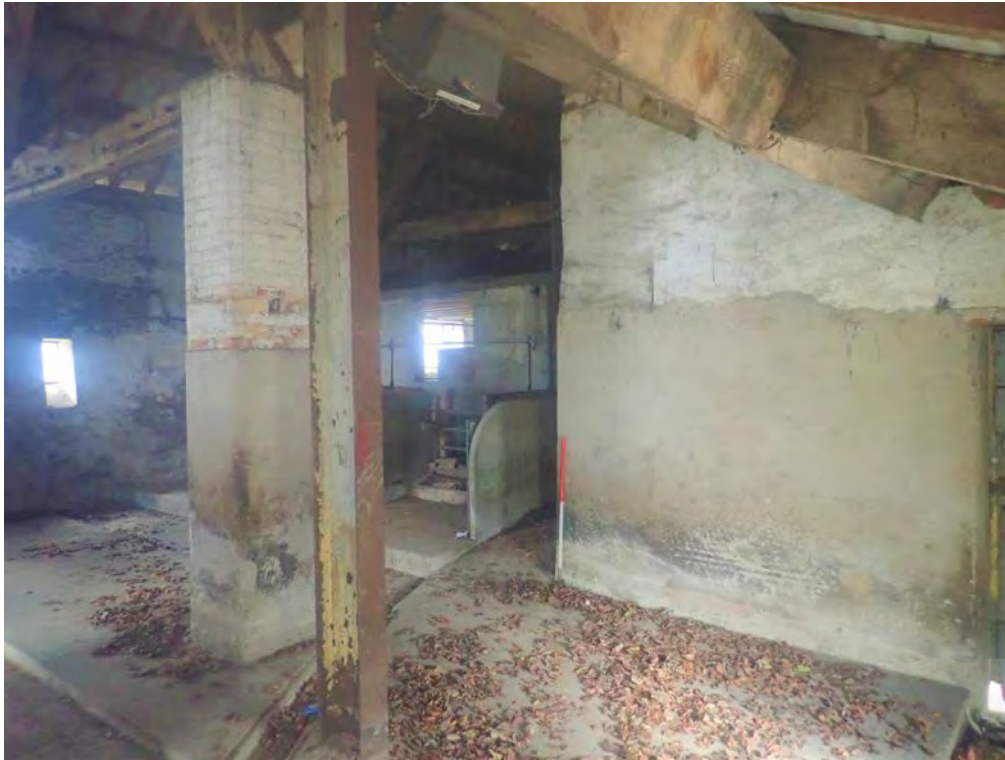
Photograph:39 Direction: N Digital Ref: NEMB2_0028 Description: NW extent of NE wall of SW outshut with steel I-beam post and brick pier to west (left).
