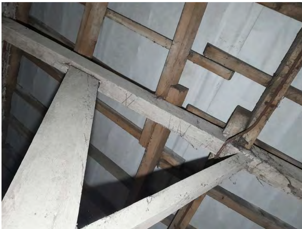
Photograph:68 Direction: N Digital Ref: NEMB2_0110 Description: Baltic marks in rafter soffit of SW truss of NE outshut.
