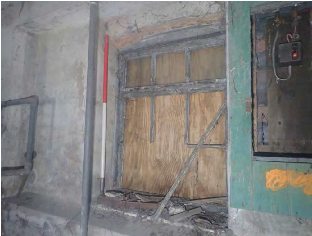
Photograph:41 Direction: W Digital Ref: NEMB2_0056 Description: Detail of partially blocked cart door to window in NW wall of Bay 2.
