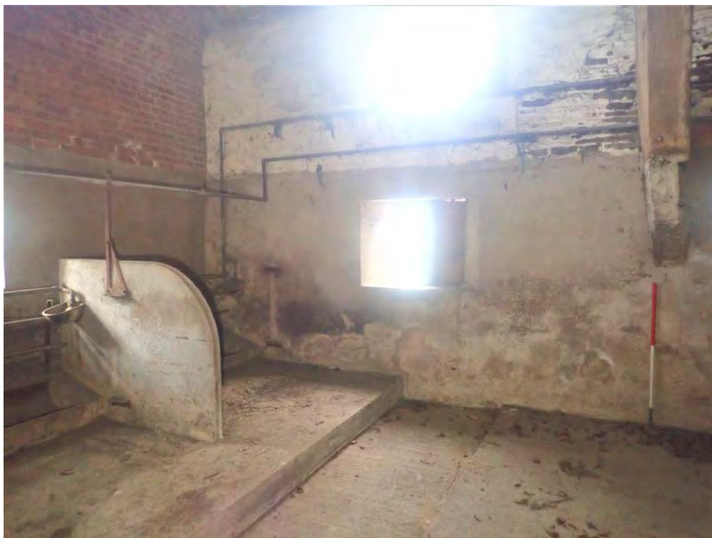
Photograph:42 Direction: W Digital Ref: NEMB2_0034 Description: West corner of Bay 1 with brick SW wall and stone NW wall with no evidence of fireplace.
