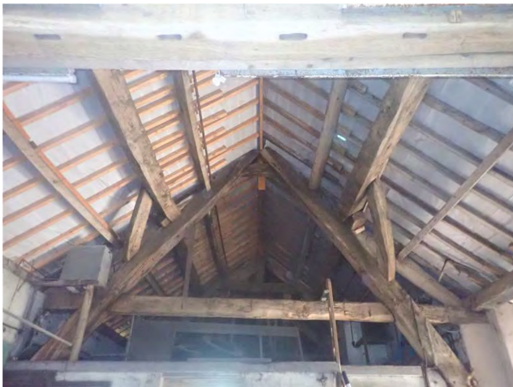
Photograph:36 Direction: NE Digital Ref: NEMB2_0073 Description: General view of SW face of Truss 2 with Truss 3 in background.
