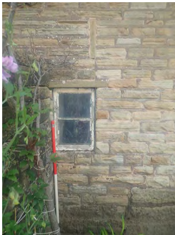
Photograph:19 Direction: SE Digital Ref: NEMB2_0015
