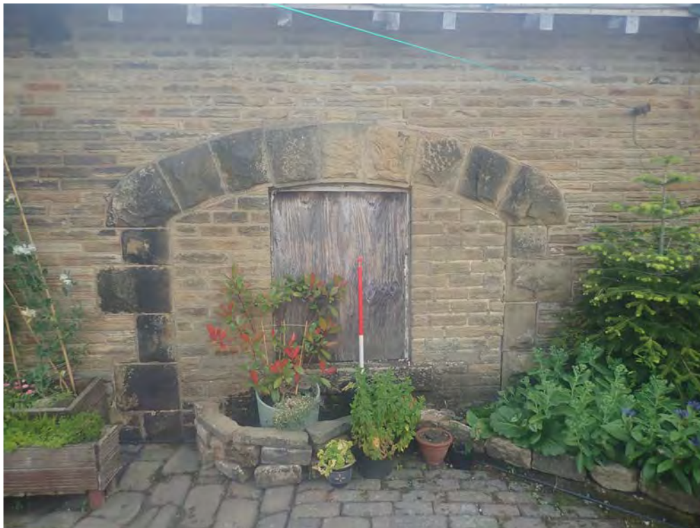
Photograph:8 Direction: SE Digital Ref: NEMB2_0014
