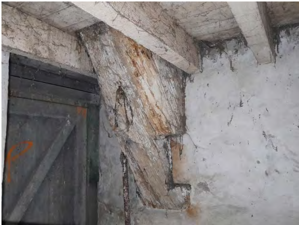
Photograph:28 Direction: W Digital Ref: NEMB2_0090 Description: Detail of Truss 2 NW cruck blade from wall and through loft floor with door in background (left).
