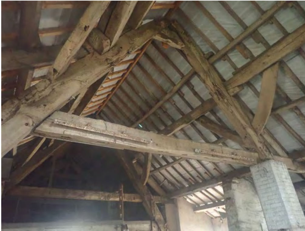
Photograph:35 Direction: E Digital Ref: NEMB2_0070 Description: General view of SW face of Truss 1 with Truss 2 in background.
