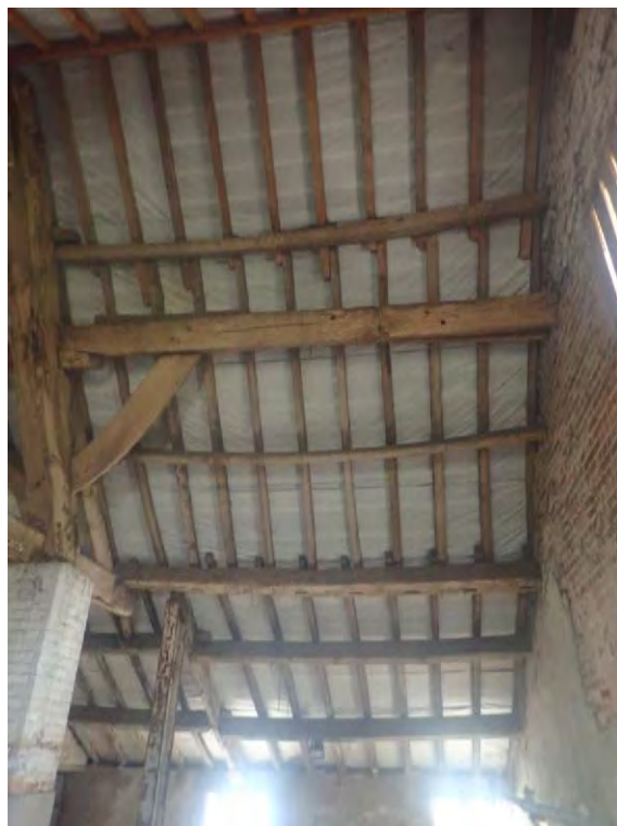
Photograph:33 Direction: SE Digital Ref: NEMB2_0071
