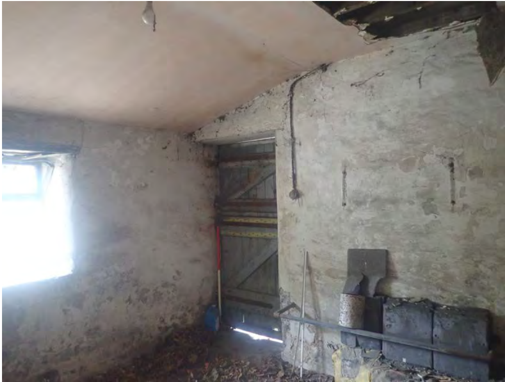
Photograph:69 Direction: S Digital Ref: NEMB2_0112 Description: Doorway in SE extent of SW wall of the NW outshut (Area E) with timber lintel.
