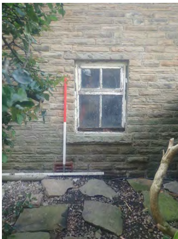
Photograph:18 Direction: SE Digital Ref: NEMB2_0011
