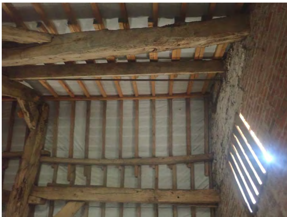
Photograph:34 Direction: SE Digital Ref: NEMB2_0072
