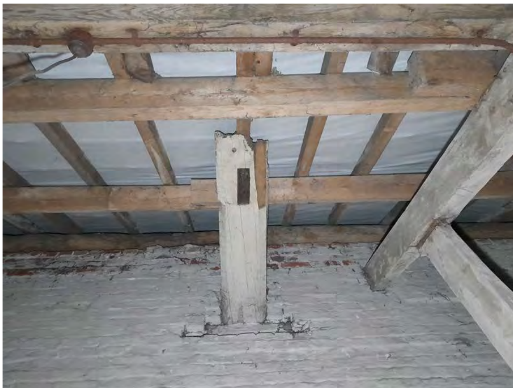
Photograph:52 Direction: NW Digital Ref: NEMB2_0108 Description: SE extent of Truss 4 tie beam with single mortice in soffit extent indicating former post.
