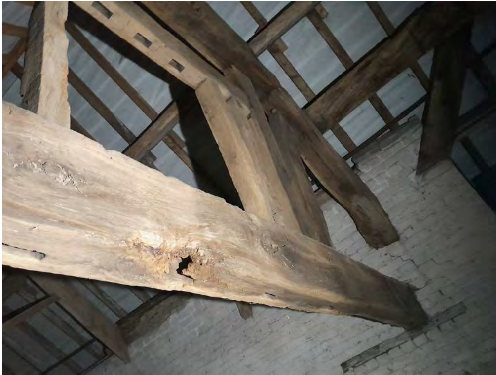
Photograph:51 Direction: E Digital Ref: NEMB2_0129 Description: General upward view of SE side of SW face of Truss 3.
