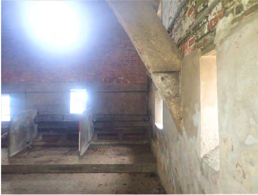
Photograph:27 Direction: SW Digital Ref: NEMB2_0032 Description:Mortice of former rail in NE face of Truss 1.
