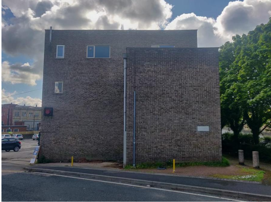
Photograph 3: Elevation presented to Lower Castlereagh Street
