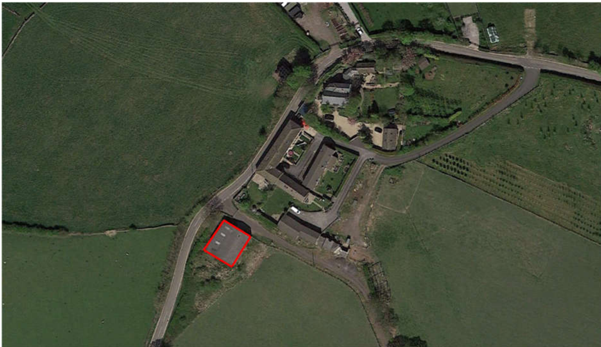
Fig 01. Aerial View of the site showing the proposed change of use building edged in red.
