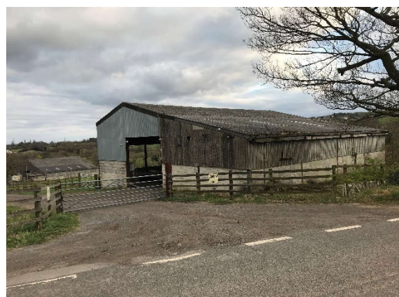
Fig 03. NE / NW elevation from South Lane
