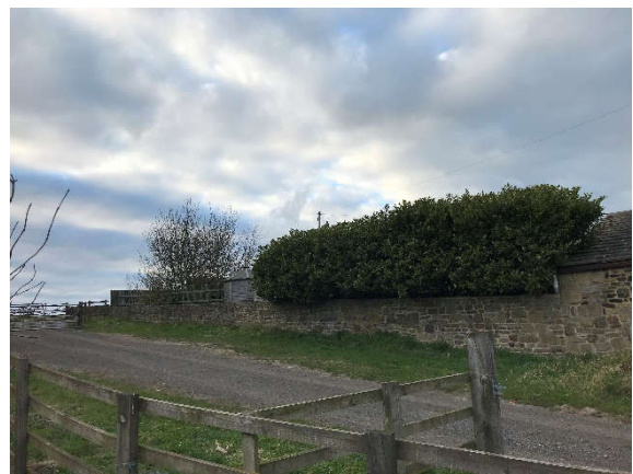
Fig 15. View of NE boundary to listed barns
