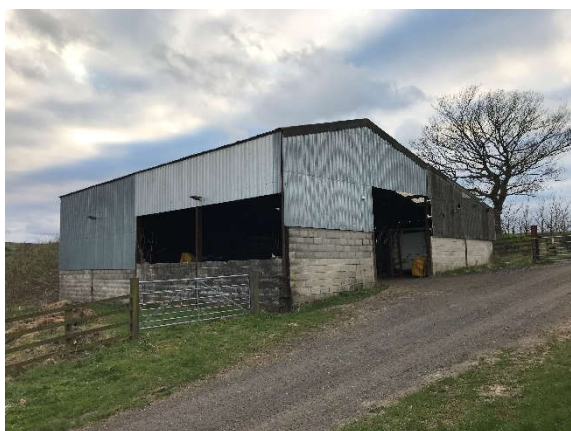
Fig 04. NE / SE elevation from access track
