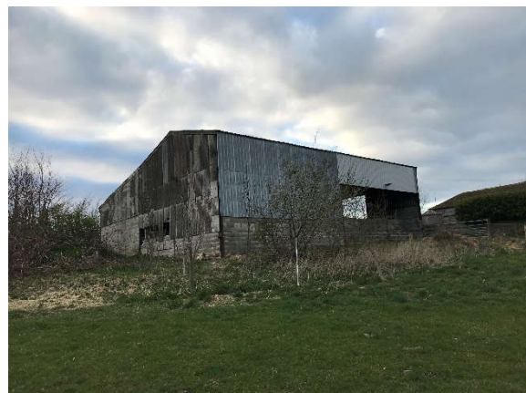
Fig 05. SE / SW elevation from field
