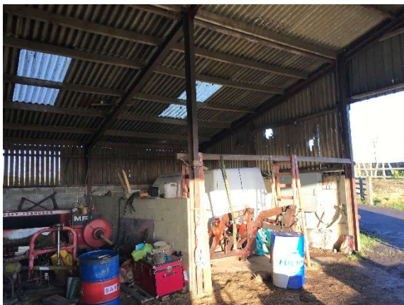
Fig 08. Internal view looking north
