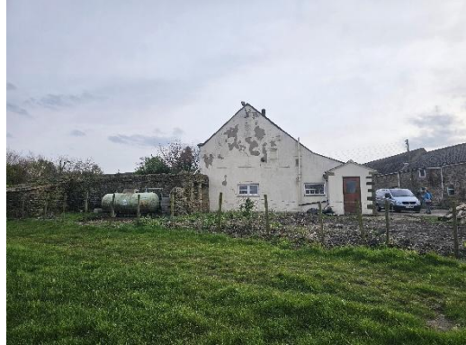
Photo 2 North east aspect Building 1
