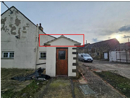
Photo 5 Gap along the verge for the porch
