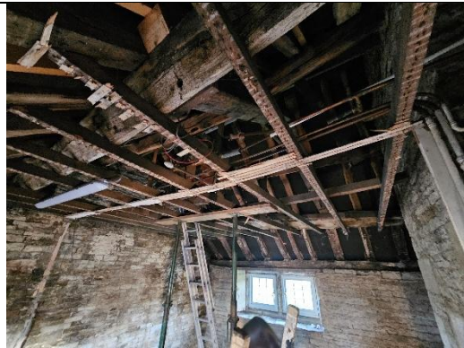
Photo 4 Internal area (the ceilings have been removed)
