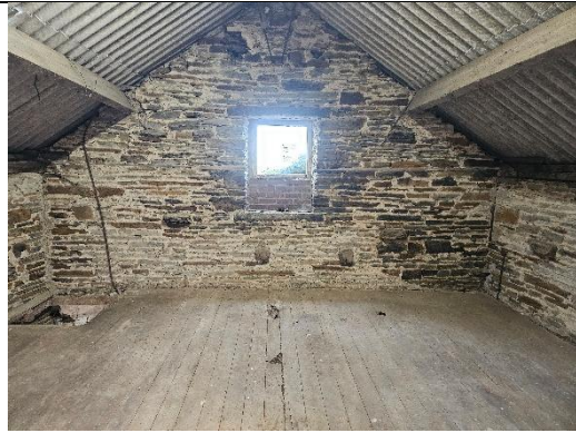
Photo 28 Internal second story Building 4
