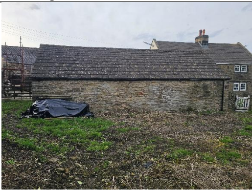
Photo 9 South east aspect Building 2
