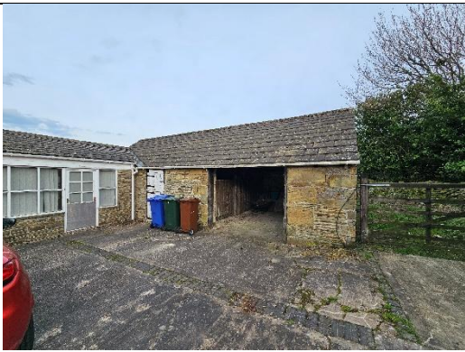
Photo 11 West aspect Building 2
