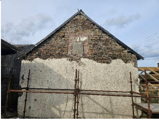
Photo 23 South aspect Building 4
