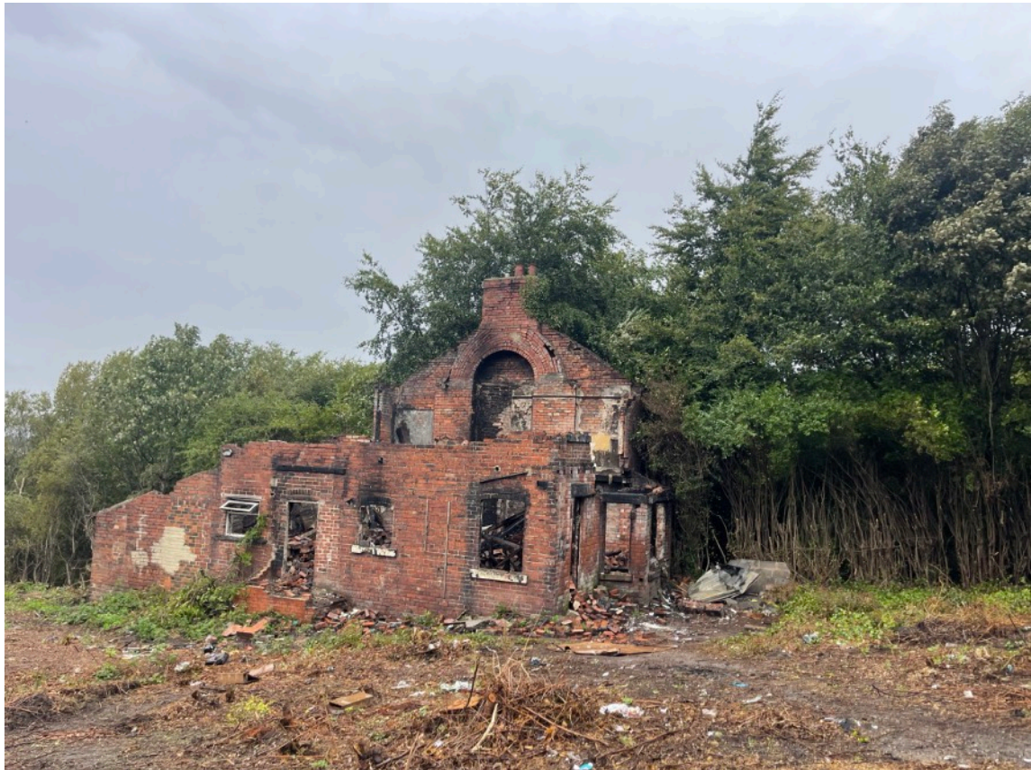
Figure 13. Derelict building with trees to the rear.
