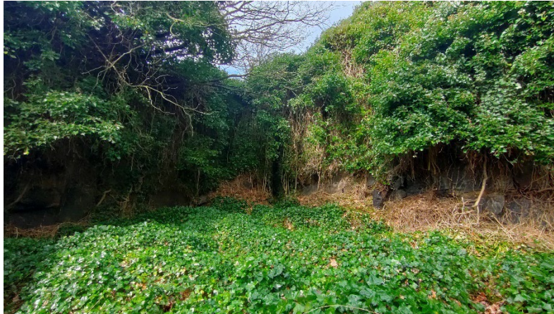
Figure 5: Inland rock, heavily covered in vegetation. Poor condition.
