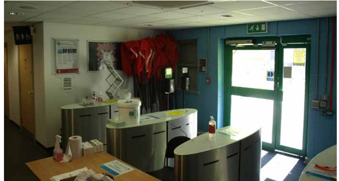
Photograph of existing entrance lobby into building
