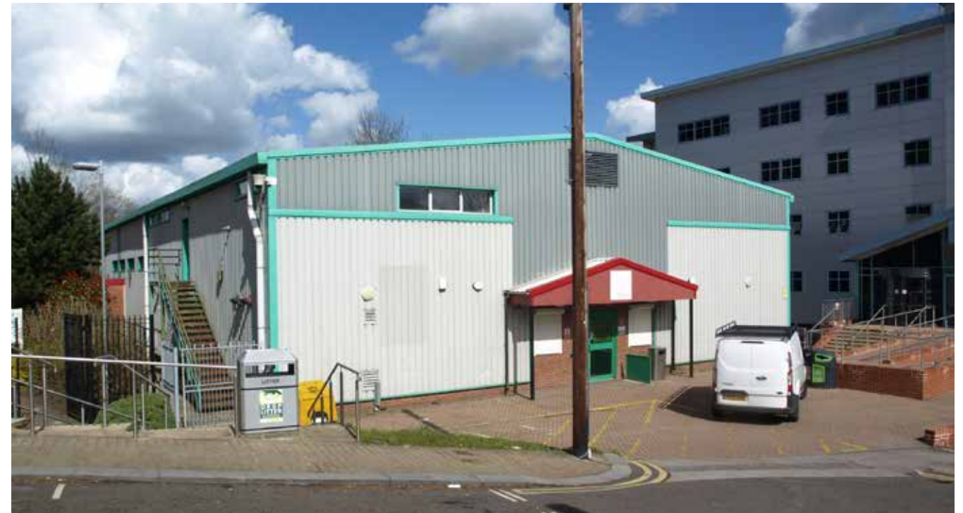
Photograph of Barnsley College Electric Theatre from Falcon Street
