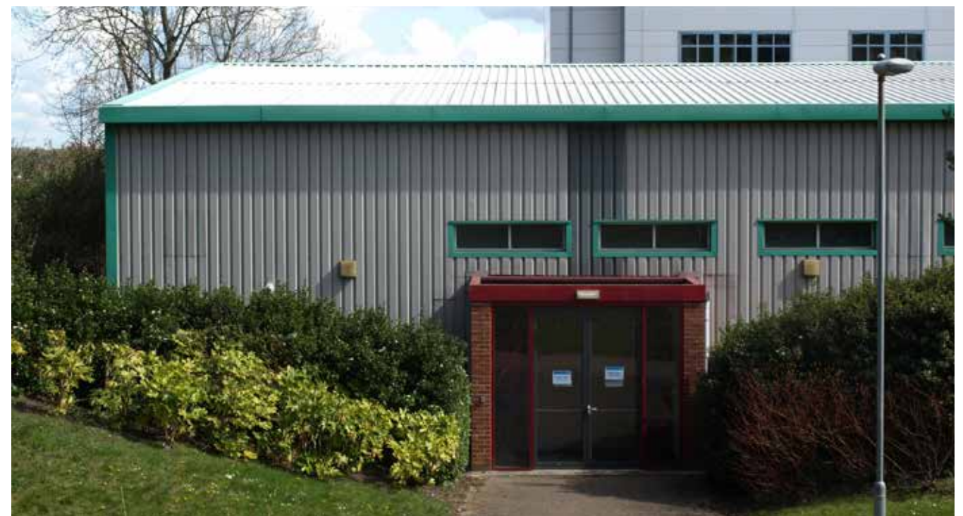
Photograph of East Entrance of Electric Theatre from Old Mill Lane Building
