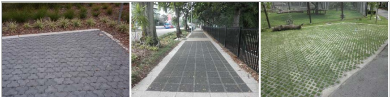
Figure 6-6: Various permeable paving surfaces
