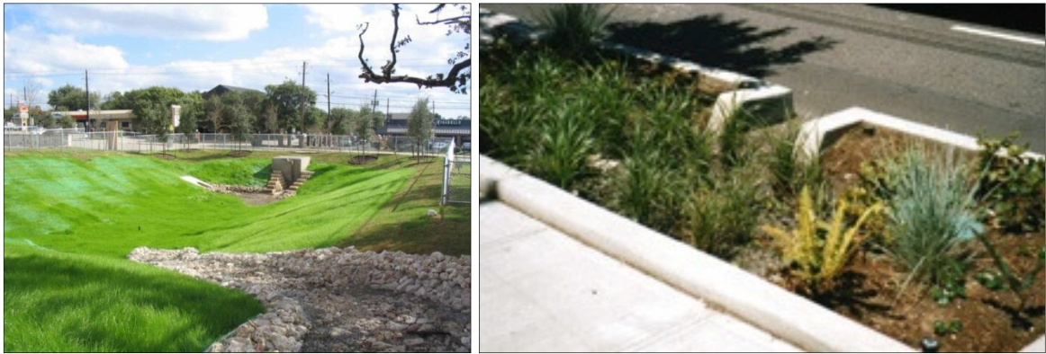
Figure 6-3: Large basin (Left) and micro storage basin (right)
