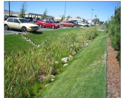
Figure 6-5: Indicative one way cross fall design (left) and constructed vegetated swale (right)
