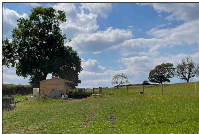
Existing Stabling on Southern Field Boundary
