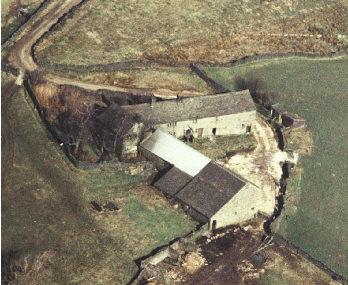
Overhead view of farmstead prior to western “lean-to” alterations.
