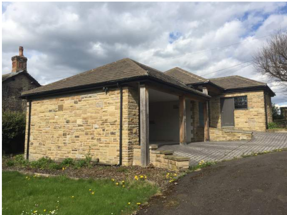
Fig. 06 – Photo of Existing Garage from the south west
