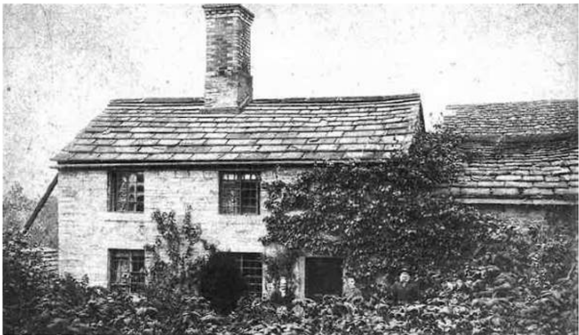
Fig 22 - Photo of front elevation of 2 Hill Top c1880
