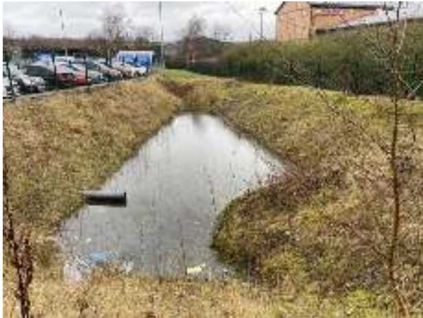
Photograph 1 – Attenuation Pond 1
