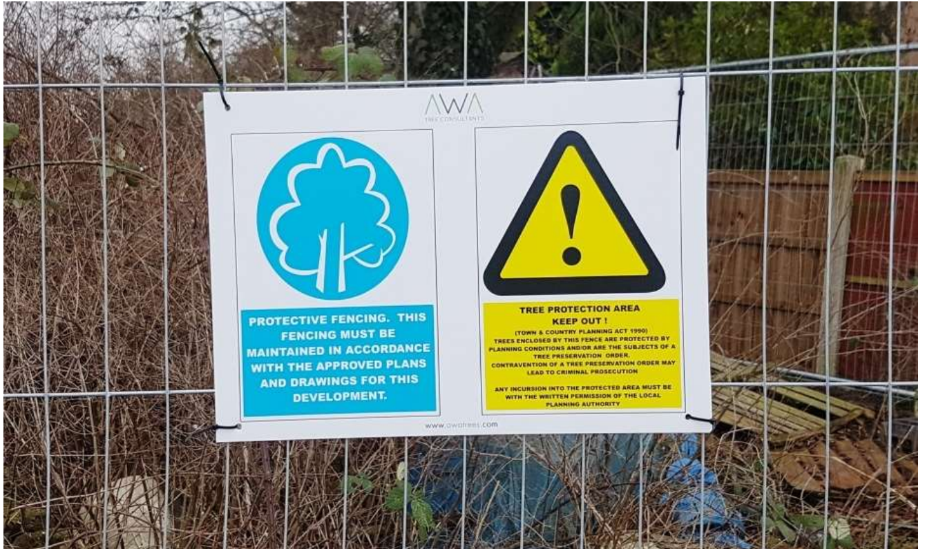
Figure 2: Example of A3 correx tree protection warning sign fixed to fencing panel
