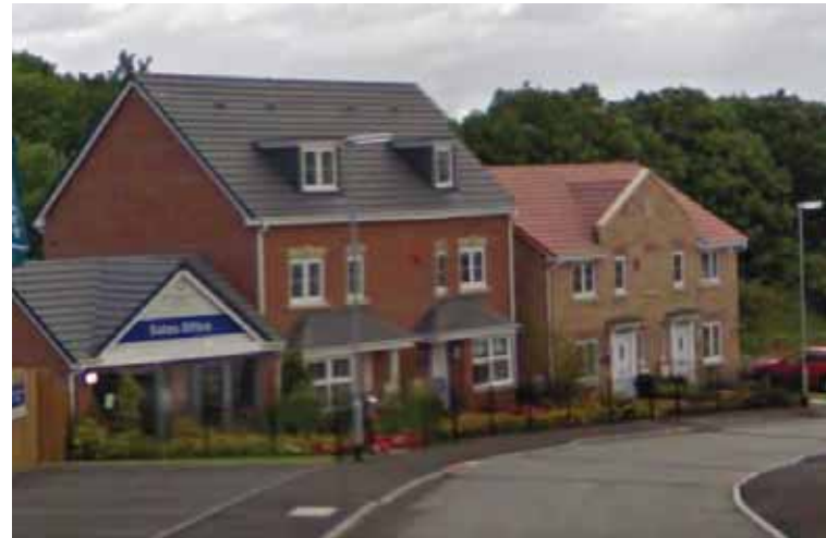
Above: Range of materials used in the wider development
